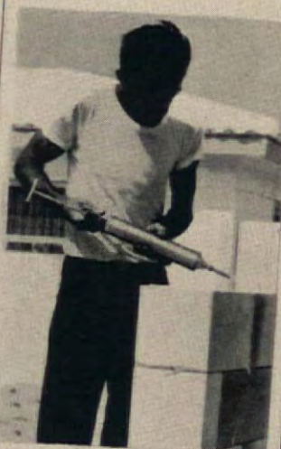
Ribbon of epoxy mortar is applied along block edges.
