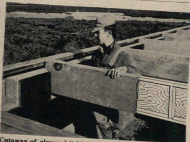
Cutaway of plywood “skin” shows 2x4” frame, stiffener.
