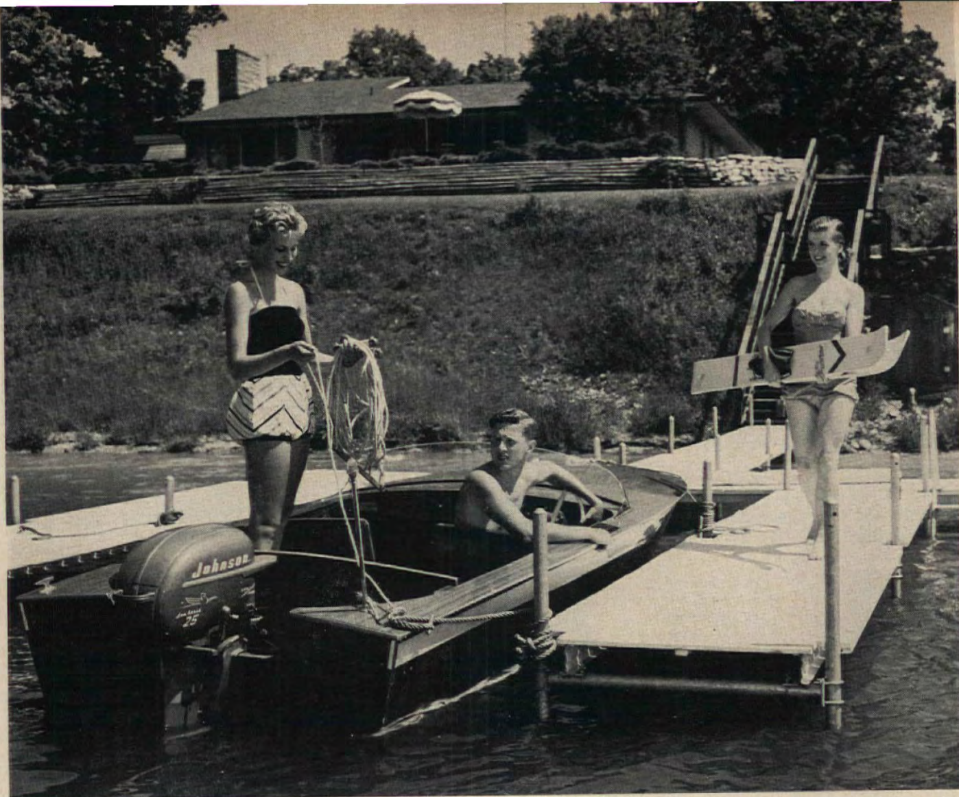
PREFABRICATED DOCK has framework of steel. Units are easily assembled and with them you can build a dock of almost any shape or size.
