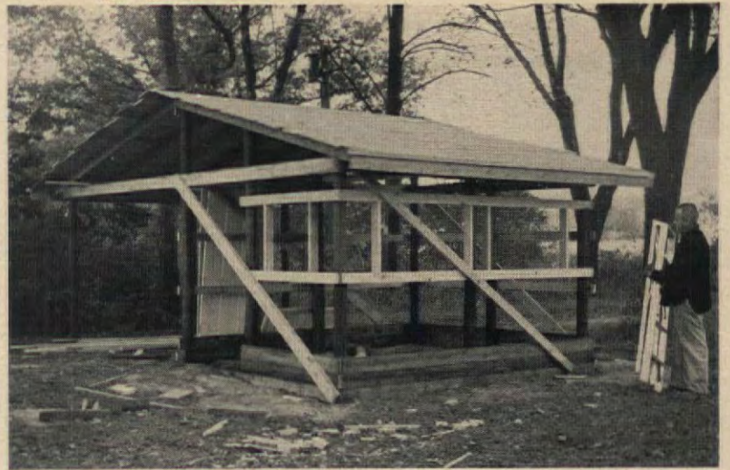
2. RAFTERS, ROOF SHEATHING and preservative-treated bottom girts are fitted and nailed in place (see sketch below). Tops of poles are sawed off level with rafters; 1x6" fascia is nailed to rafter ends.
