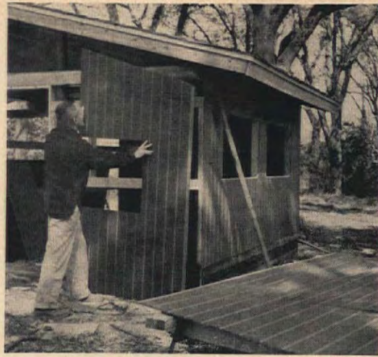
4. GROOVED HARDBOARD SIDING in 4x8' sheets can be installed quickly. After cutting roof slope hold panel in place to mark window openings.
