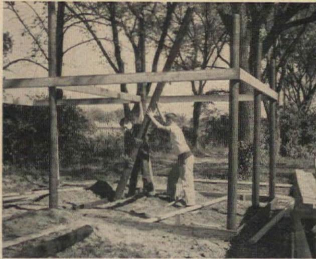
1. BASIC FRAME of preservative-treated poles and 2x6" top and bottom girts support carport-tool shed. Corner poles must be plumbed straight, braced diagonally to girts.
