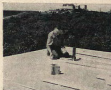
Next come sills, joists, and subfloor. Right: rough interior shows block chimney, and bare stud walls.
