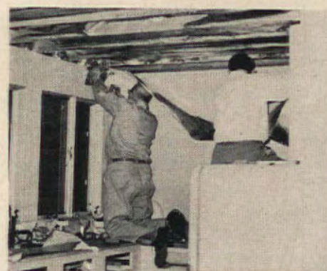
Mr. Mason staples reflective insulation between ceiling joists in kitchen. Next: furring, acoustic tile.
