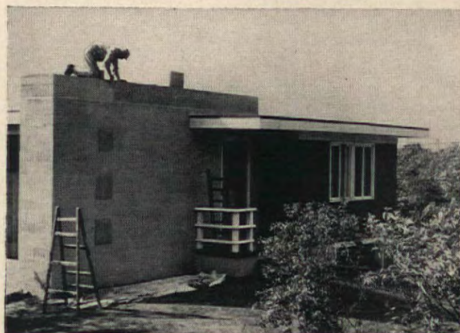
Almost done: concrete cap is troweled over the top of the chimney to keep water out of chimney blocks.
