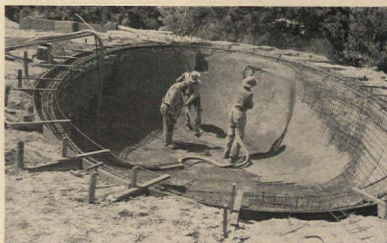
BLOWING CONCRETE under high pressure over, around steel reinforcing mesh in excavation makes "gunite" pool. No forms needed to hold concrete.
