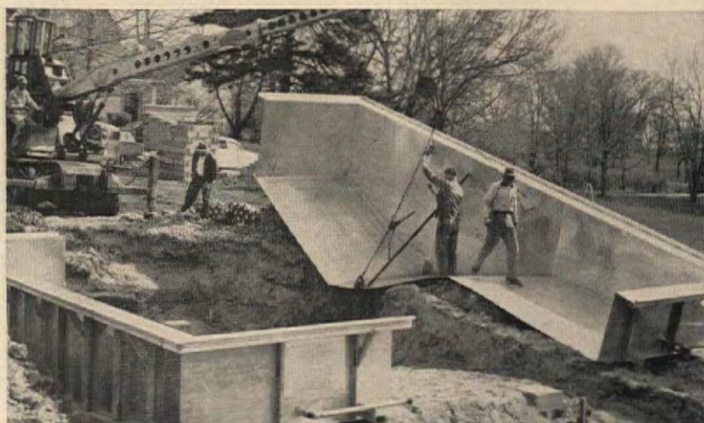
METAL POOLS are popular. This aluminum model arrives in two lengthwise sections ready to fit into the ground. Notice pipe connections are installed.
