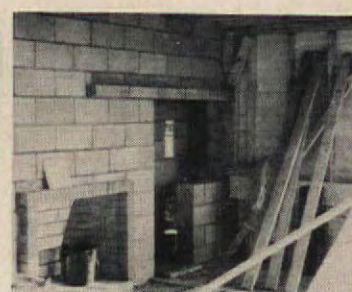
Next come sills, joists, and subfloor. Right: rough interior shows block chimney, and bare stud walls.
