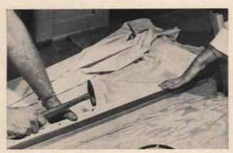
6. Couch is upholstered in 2 layers of fabric, muslin and upholstery. Remove back. Double-fold 2" of muslin, place under front edge of seat frame. Slip cardboard strips between folds to keep fabric from pulling between tacks. Tack along underside of seat frame, from center out to sides.
