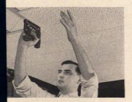
can easily install a Cushiontone sound-condiing ceiling. The handy 12" x 12" or 12" x 24" are quickly stapled, nailed, or cemented over or cracked plaster. Cushiontone can be reted without loss of noise-quieting efficiency.
