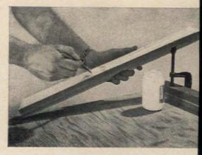
1. Cut plywood seat and frame parts as diagrame Glue and clamp frame edges to seat. Turn seat ove drill and countersink five holes in front and bac three in each end, and screw top to frame with 1½ screws. Drive 2" brads across mitered corners.
