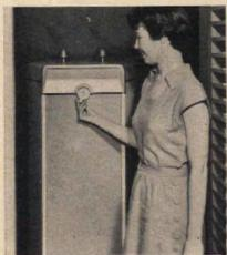
Water heater, hidden behind decorative louvered doors in its own specially designed closet, is conveniently close to sink and laundry area. Controls are placed so that they are easy to reach and to read whenever special adjustments are necessary, and they are above the reach of small frys' exploring fingers. Glasslined heater, smartly styled in turquoise, blends with the rest of decor.
