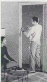
Screw clips to door jamb
