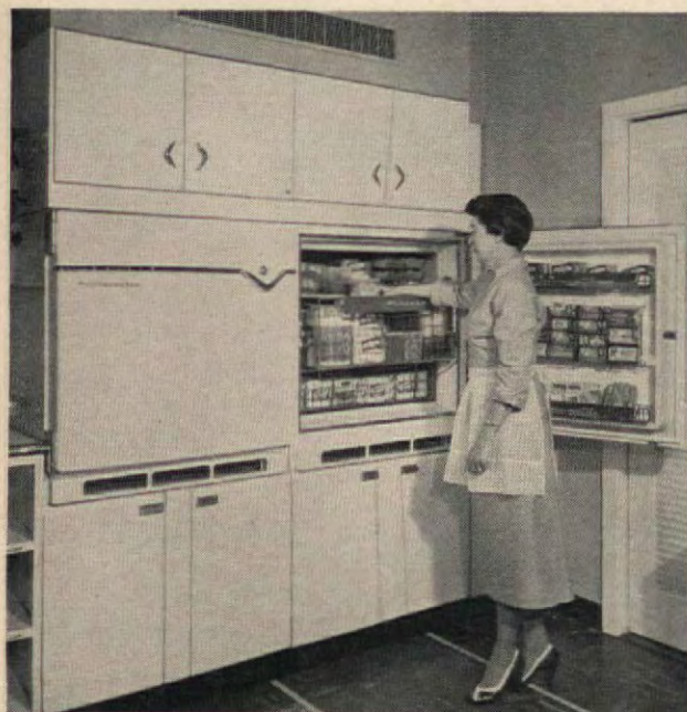
Work-level refrigerator, freezer each have own cooling system. Cubes in freezer; freezer supplies in cabinets top, bottom.
