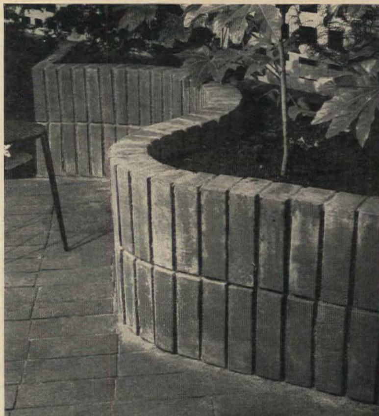
Serpentine wall for raised bed is two bricks high, only one brick deep, but curved shape gives strength. Designed by Donald Gutoff, landscape architect.
