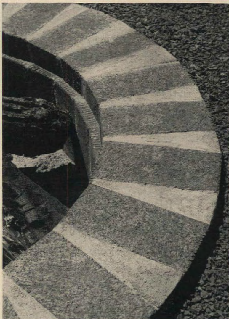
Bricks laid flat around circular firepit are separated by wide mortar joints that help form "radiating" pattern. Designed by Crawshaw and Polleccek.
