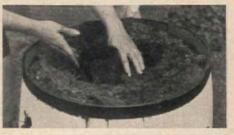
With a spike, punch holes along its length (after filling it with sand to avoid denting it). Set barrel on firm base, put 3" of gravel in bottom, stand pipe in center, and support it while you . . .
