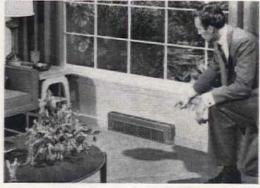
Exclusive blenders are the secret of the Blend-Air system. Unlike ordinary registers, Coleman blenders pull room air in and mix it with fresh, cool air in summer—or with heated air in winter. Keeps temperatures even, floor-to-ceiling and wall-to-wall. NO drafts, ever!
