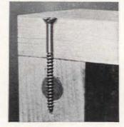
Before driving screw into end grain, drill hole lengthwise through board and glue in dowel as shown. Makes a strong joint
