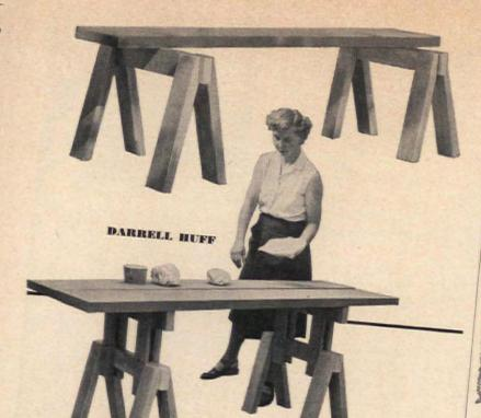
Fasten tapered legs to 24"-long 2 x  $4\rm ^{\circ}s$ screws on each. To make extensions, screw four pieces of I x 4 one inch from ends, using glue and three to remaining two 2 x 4's, 4%" from ends as shown. Drill 1/4" holes through these 1 x 4 legs, 6" from the bottom of each leg. To use extensions to raise horses, slip a 20 penny spike through holes and set extensions on top of the horses
