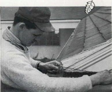
Tired of semi-annual gutter cleaning? Then build these leafproofers. First clean gutters. Then cut 1/3" galvanized hardware cloth into strips an inch wider than gutters. For wooden gutter, nail screen to one edge. For metal gutters, staple screen to roof under first row of shingles, or bend up small lip along screen edge and staple to side of house. Overlap all joints
