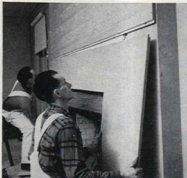
6. Cut lower panel to fit around fireplace facing. Because existing marble here was handsome, it was retained. Put rabbet in top of panel and bring panel up to make a close fitting joint with top panel. Secure in same way as top panel
