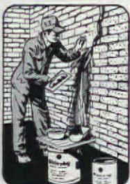
Scoop up fast-setting WATER-PLUG on trowel, and
