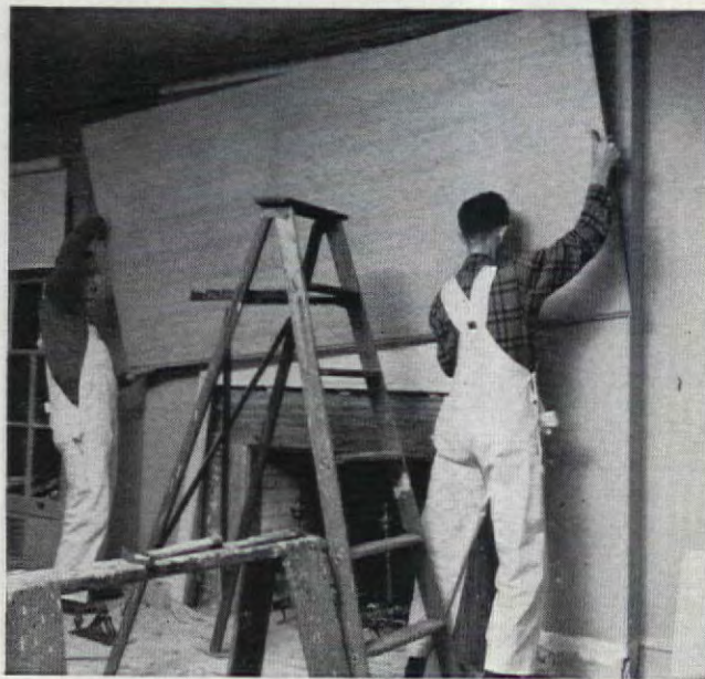
3. Cut \frac{3}{4} -in plywood to size of fireplace. Place sections on wall horizontally to eliminate vertical joint centered directly over fireplace opening. Meeting edges of panels are rabbeted to produce half-lap joint, with rabbets \frac{3}{8} in. deep, \frac{3}{4} in. wide
