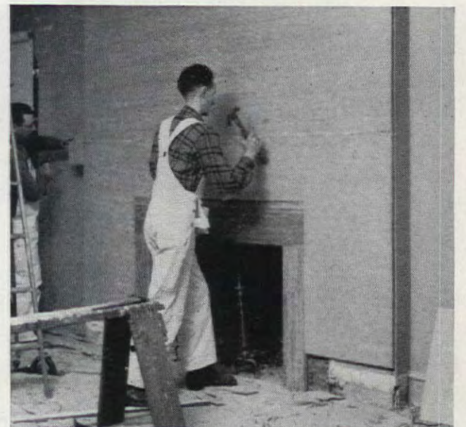
7. As standard plywood panels are 4 ft. wide, two will take care of average 8-ft. high wall. If slight gap remains at bottom, as in this case, it can be covered by a simple baseboard. If larger gap results from high ceiling, use small filler piece of plywood
