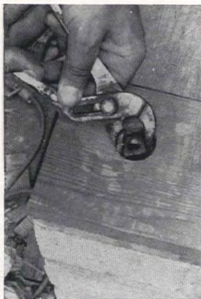
Drill through both boards a hole the size of bolt in center of previous hole. Bolt sills down, and if bolts project above the surface, cut them off flush with a hack saw
