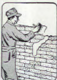
Water now sealed off. Coat wall with THOROSEAL.
