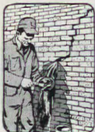
Mix WATERPLUG with water to consistency of putty.
