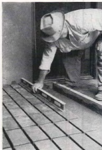
Floor was built of "split bricks." These are only half as thick as regular bricks. Bricks were laid on a bed of mortar troweled on the old floor to a thickness of one-half inch
