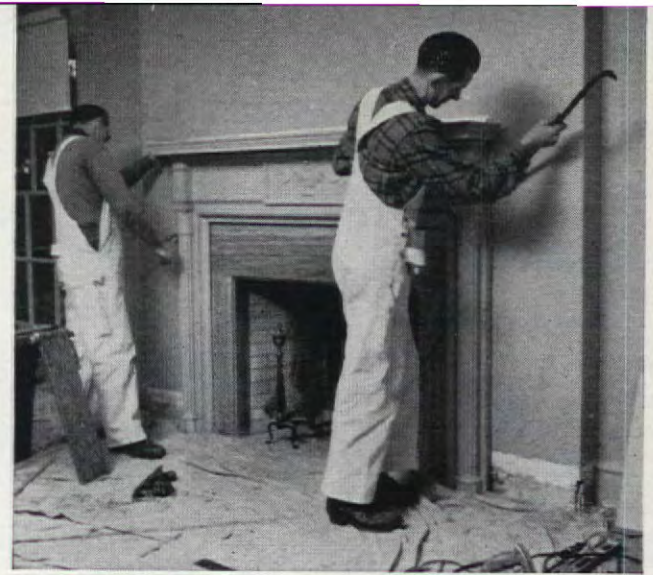
1. Remove old mantel by carefully prying it from wall with the aid of pinch bar. Insert blocks of wood between mantel and plaster to protect them from damage from bar. Try to get mantel off in one piece as you may find use for it at some later date
