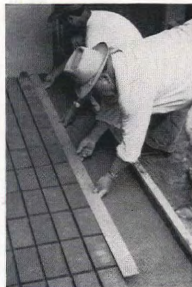
The bricks were laid on the mortar one full row at a time. For a job like this, check bricks with level and straight board for alignment. Let the bricks set overnight
