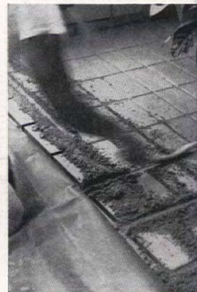
Three parts sand were mixed with one part cement and very little water, and worked between bricks. This dry mix requires sprinkling with water every 12 hours for two days
