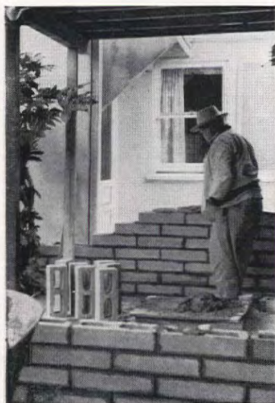
After the footings were poured, the masonry block wall was built of 4- by 16-in. blocks. Reinforcing rods were put in corners and back wall to strengthen the one-course construction
