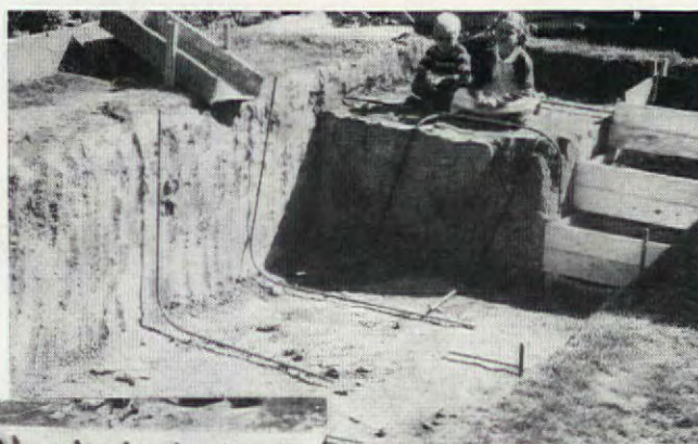
Forms can be made of scrap lumber, but must be sturdy and well braced on both sides. Below ground level, dirt walls serve as outer form; above that, provide plenty of reinforcement
