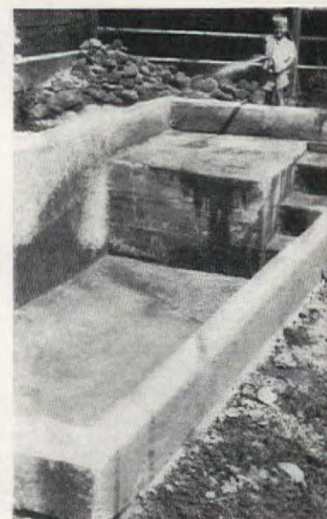
Excavation finished, steel reinforcing rods, bent by hand, were held in place with heavy wire forced into the ground to anchor it firmly
