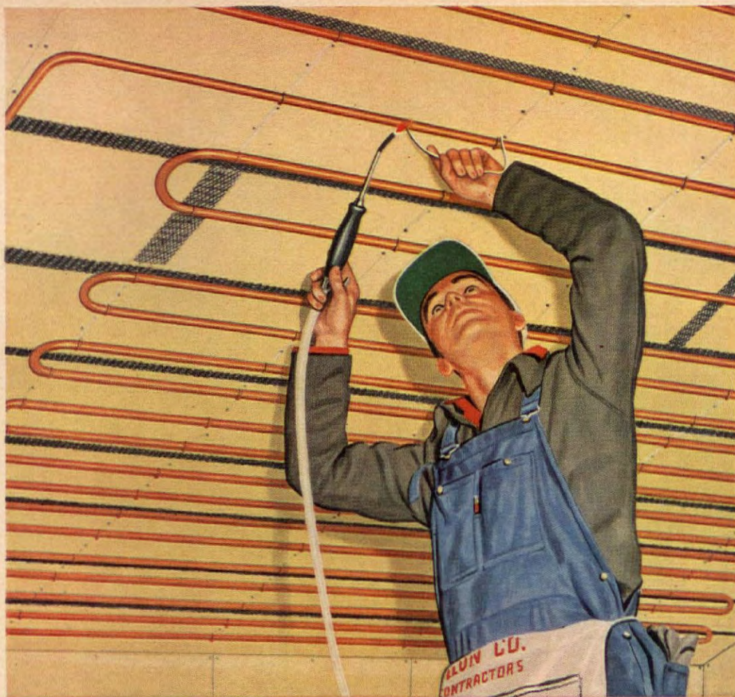
Ceiling radiant heating coils of Bundyweld® Tubing are quickly, economically installed, then plastered over to form invisible source of gentle, even radiant heat.
