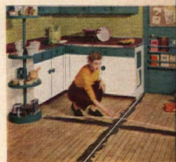
Here Mrs. Loock finds the center of the floor. Next, she'll spread Kentile Adhesive over half the floor before laying the tiles in place.
