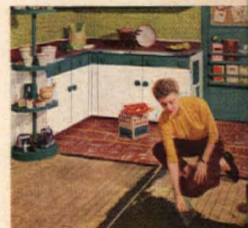
With half the floor installed, Mrs. Loock spreads Kentile Adhesive to cover remaining half. Then it's simply a matter of putting tiles in place until entire floor is completed.
