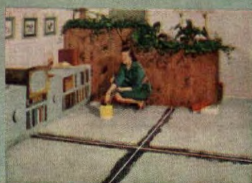
STEP 1... Mrs. Lansing follows the simple instructions. Here she's beginning to spread adhesive over half the play room.
