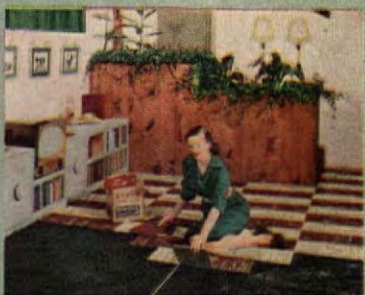
STEP 3... After adhesive is ready, Mrs. Lansing continues installing tiles... and the other half of the
