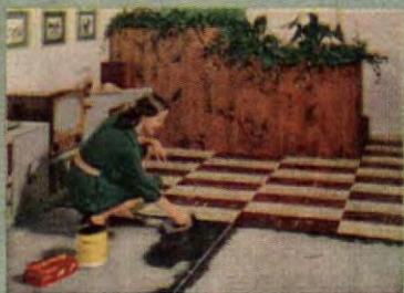
STEP 2... She puts tiles down in place, one at a time. When half the floor is covered, the adhesive is spread over the remaining half.
