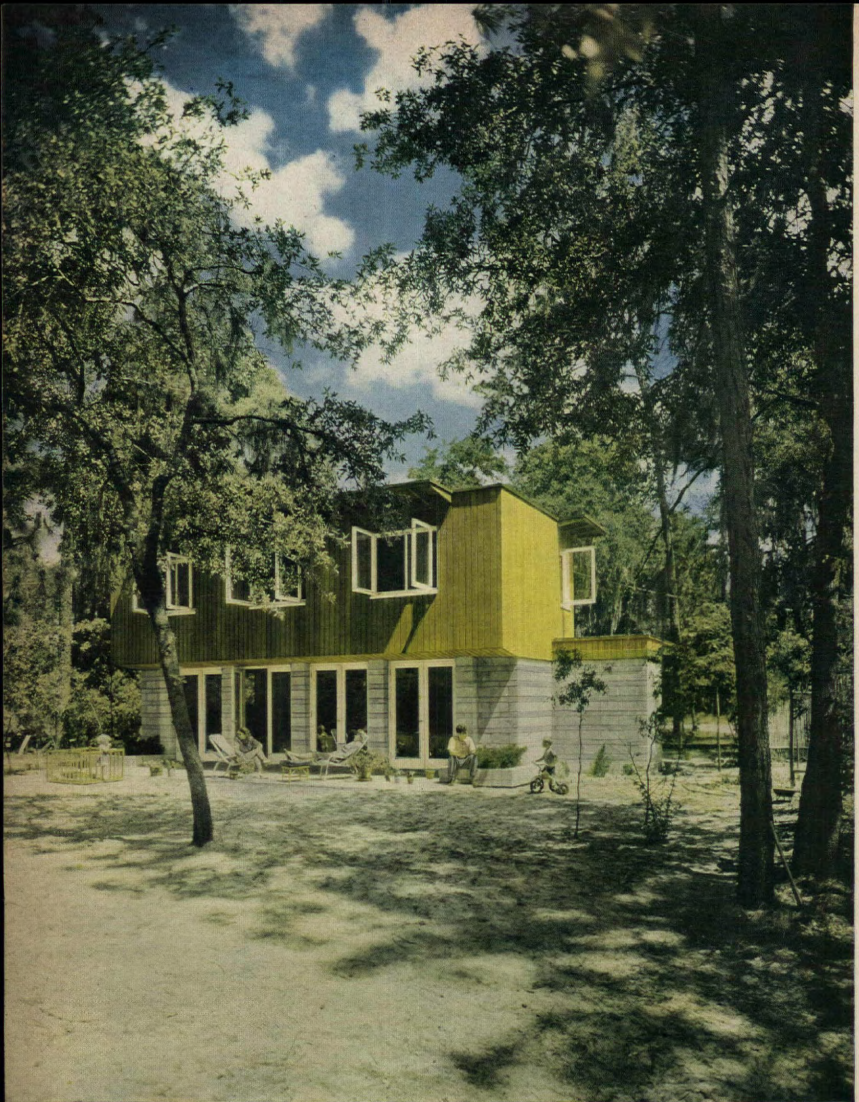
Ground floor walls are alternate courses of 4-in. and 8-in. concrete block. Upper walls are 1 x 6-in. cypress boards rubbed with shingle stain before fastening. Stain was mixed from yellow and green to approximate foliage color
