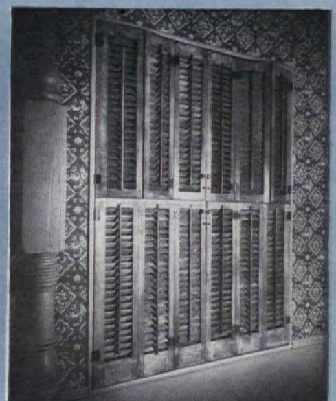
Here is a six-panel set of shutters cut through the middle. Either the top or bottom, or both, can be folded to the side, or closed to suit the light conditions at the moment
