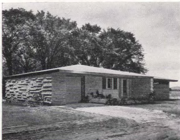
Hipped slate-surfaced roof is cemented and rolled. Wide overhang gives weather protection to front entrance and garage
