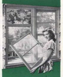
To take out, just move the upper sash down, the lower sash up. Press each window to left against spring cushion and REMOVE.
