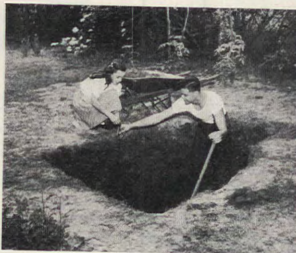
The pit is now below frost level, and ready for the three cubic yards of cinders required to provide drainage and to prevent heaving by frost
