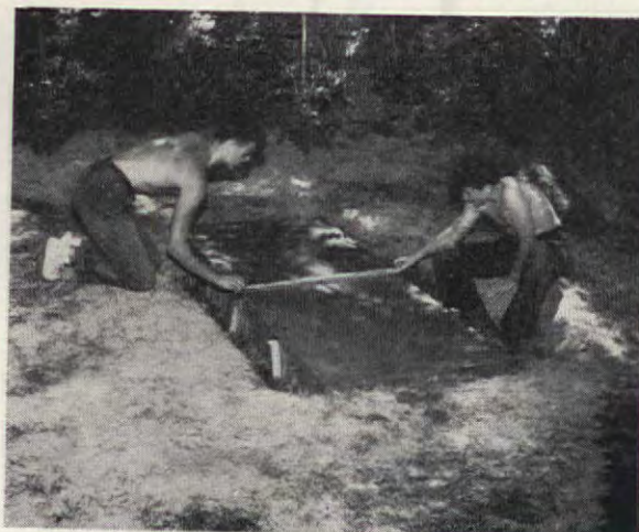
When the form is packed with cement, the surface is finished off by sliding a straight board along it, pushing off excess, and filling in depressions
