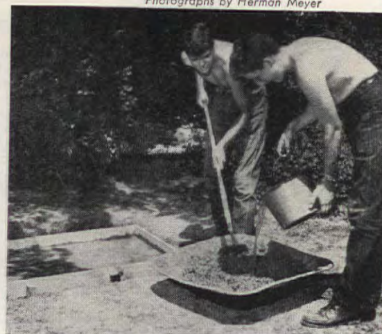
Cinders are leveled off 8" below surface, four level sides make form for concrete, stakes prevent bowing from weight of cement
