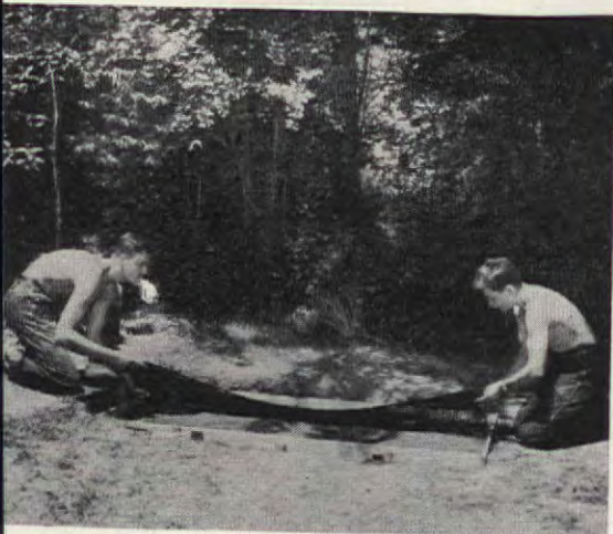
After slightly more than half the concrete has been poured into the form, a wire mesh is laid over this, and the additional cement then added
