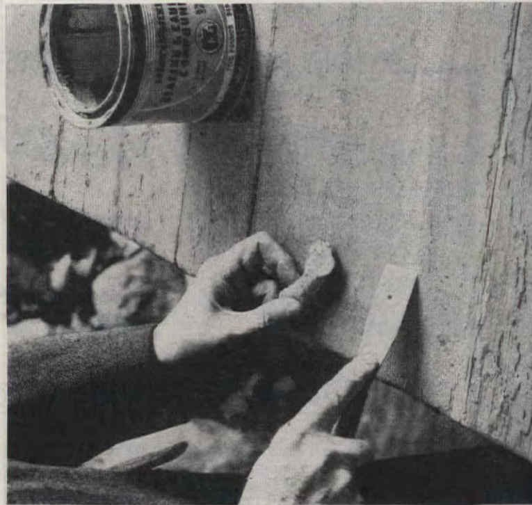
No. 6 Because they are more flexible to changes in the weather, use caulking compounds in the cracks
