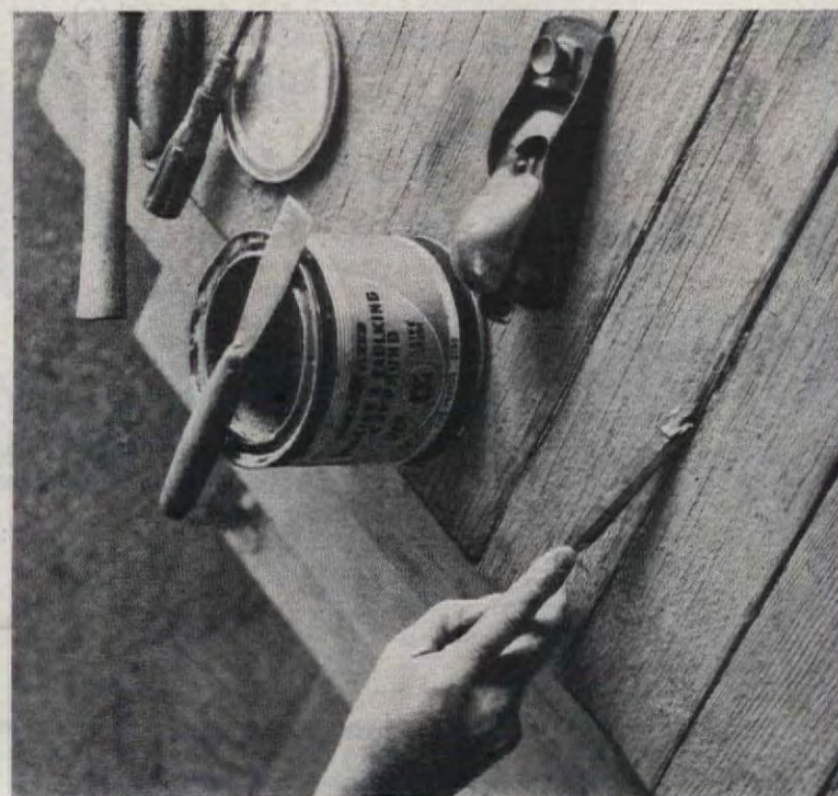
No. 4 A chisel proves handy where surface defects are minor. Splinters may be removed quickly in this way
