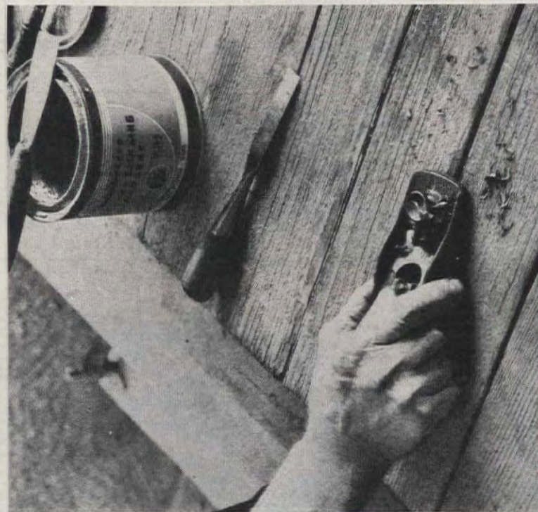
No. 5 Where surface is extremely rough, use a plane to produce clean, smooth and even working surface
