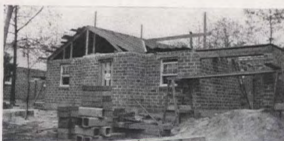
Interior partitions can be put up independently of the light-weight, concrete masonry unit walls
