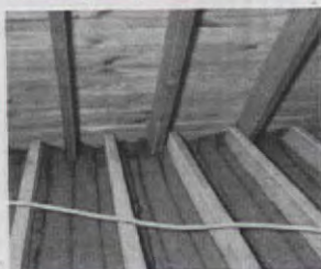
IN EXPOSED ATTIC FLOORS... A simple job. Merely expand KIMSUL; fasten at ends and sides.
