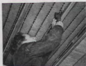
IN SLOPING ROOFS... Easy with KIMSUL. Just fasten to plate, ridge and sides of rafters.
