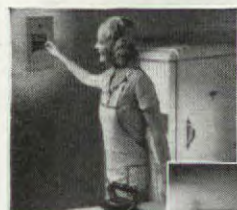
A simple movement of a lever restores current—unless danger still exists.
