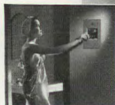
A simple movement of a lever restores current—unless danger still exists.
