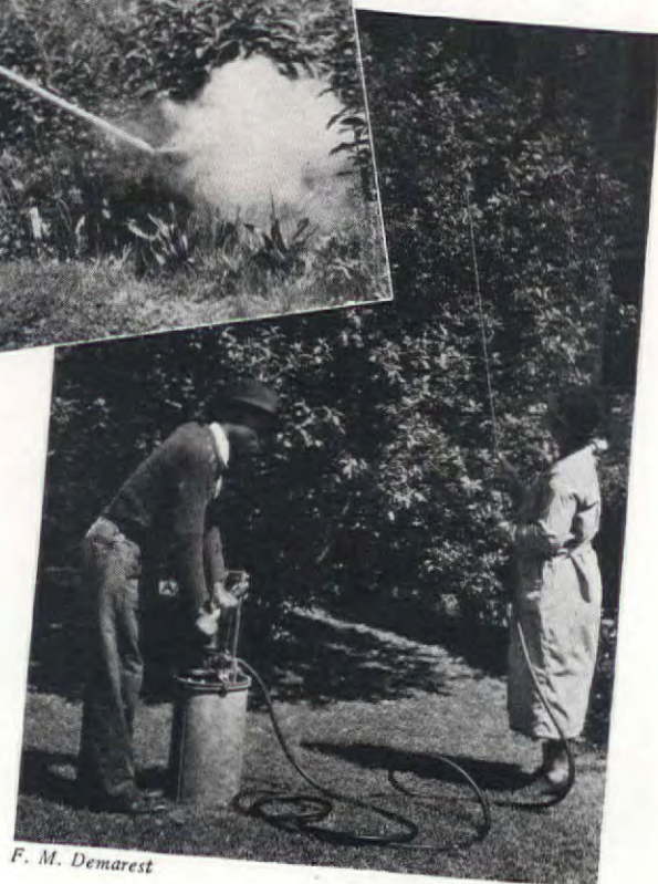
With adjustable nozzle one sprays under the lowest leaves with ease
