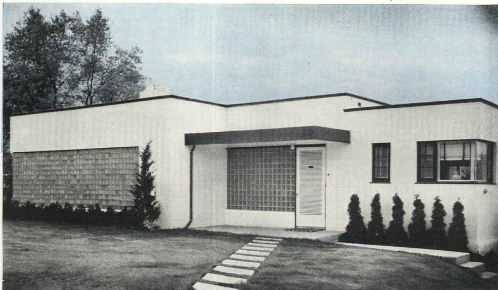
Front entrance detail and exterior walls of glass block in hall and living room
