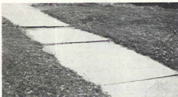
Water unable to escape through a poorly drained lawn area may freeze and throw flags out of line
