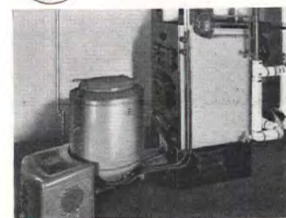
Mr. Reese's hot water heating plant and the Iron Fireman which provides automatic self-regulating firing.
