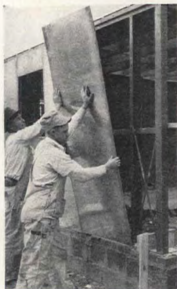
The walls are made of copper plates held together by a special extruded shape which is bolted firmly to the steel framework
