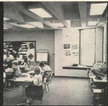
The classroom window (above and drawing) sharply reduces sound entering the classroom from play spaces just outside (left). Sound transmission from room to room is slight, and room-to-room view is cut off by projecting duct enclosures (which also house pipes, vents, and roof drains).
