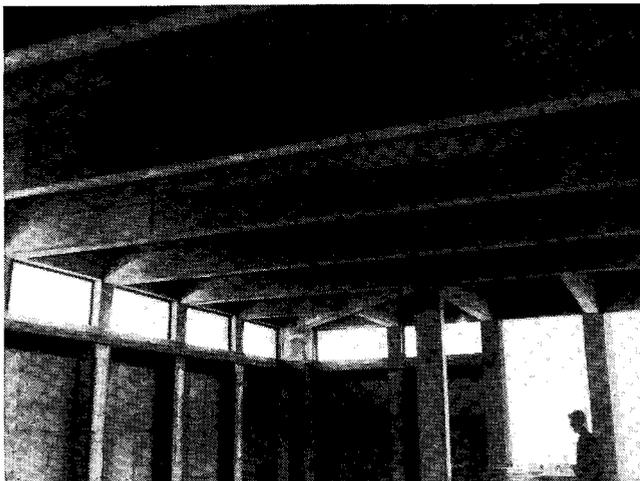
(7) Cast-in-place beams over the recreation area of the building are post-tensioned.
