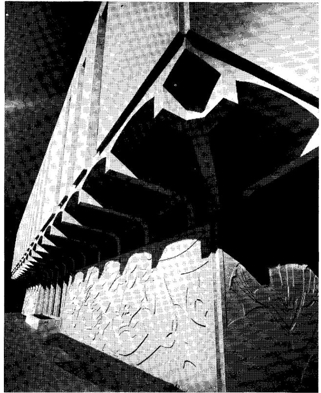
(8) West facade of building features sculptured, cast-in-place exterior walls. (9) Precast panels are used for walls above first floor levels.
