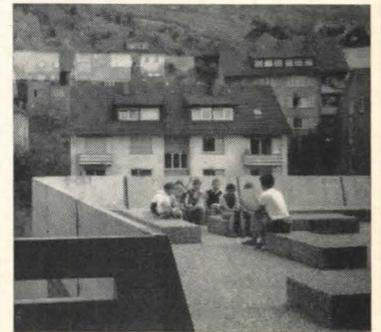
Much of the structure of the building is poured-in-place retaining walls, columns, beams, and ceiling slabs. The deep exterior parapets and fascias, however, are of precast concrete; and interior partitions are of face brick. The pleasant contrast between the roughly formed, poured-in-place surfaces and the smoothly precast parapets is one of many subtleties in detailing.
