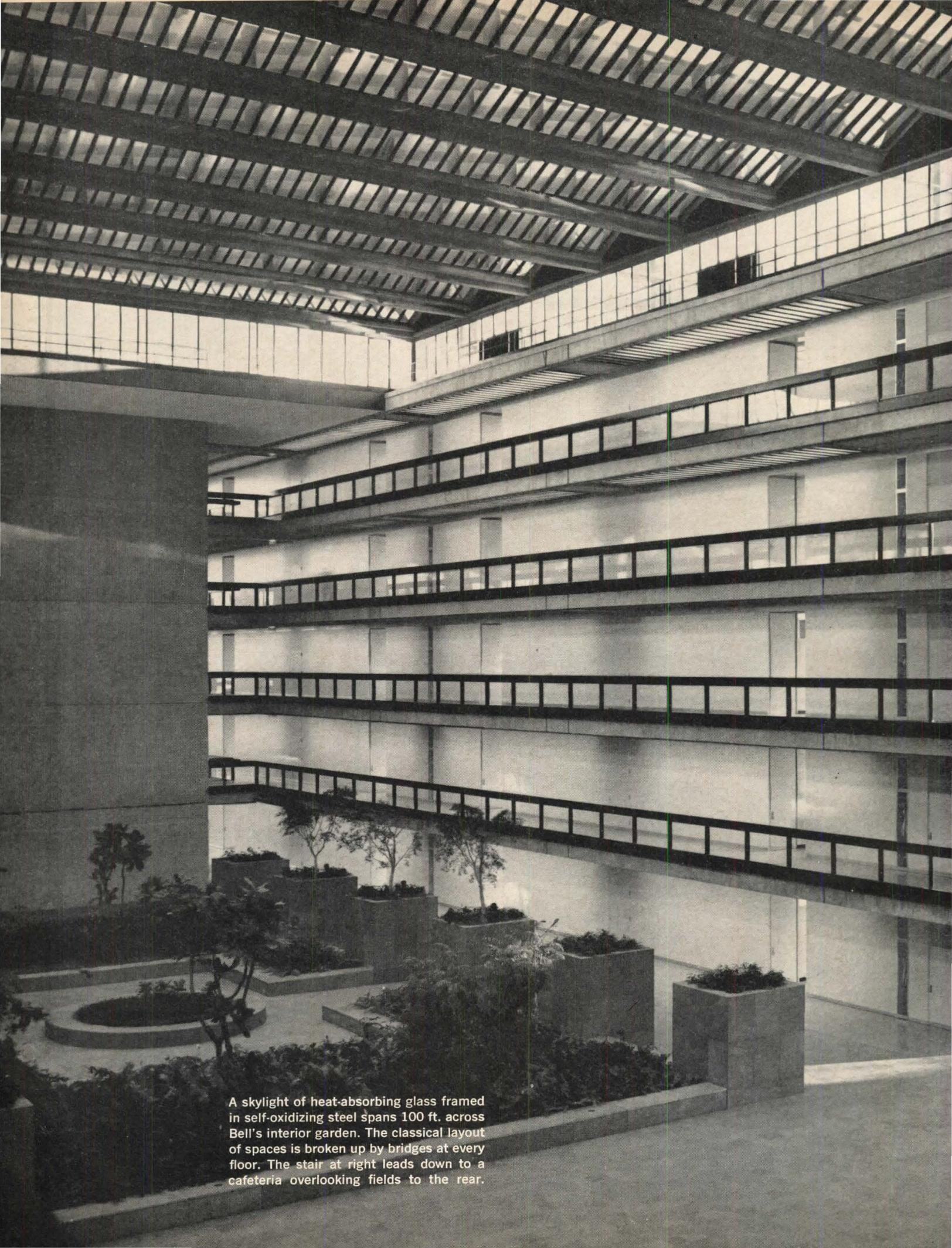
A skylight of heat-absorbing glass framed in self-oxidizing steel spans 100 ft. across Bell's interior garden. The classical layout of spaces is broken up by bridges at every floor. The stair at right leads down to a cafeteria overlooking fields to the rear.
