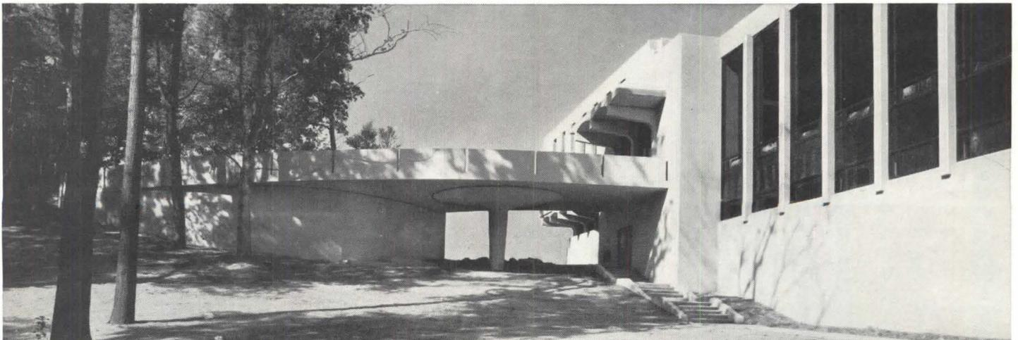
(2) Cast-in-place, post-tensioned entrance bridge takes advantage of the terrain. Bridge was cast integrally with the giant *mushroom* base. (3) Precast columns are used
