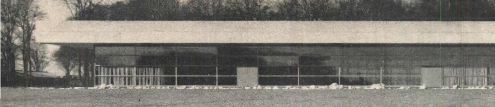
double-columns of steel; these double-columns, placed 60 feet on centers, carry primary trusses in the short direction of the roof; they have a 120-foot clear span and they cantilever another 30 feet or so beyond the columns at each end.
