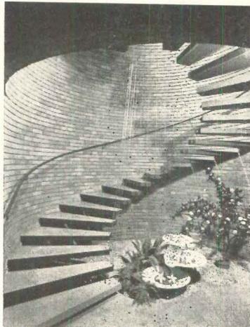
ended circular stair (above) was added inside, leading gracefully to the office floor. Luminous ceilings were originally planned for the office area (right). But, when the city required sprinklers, the additional \$9,000 expense was met by shifting to strip lighting.
