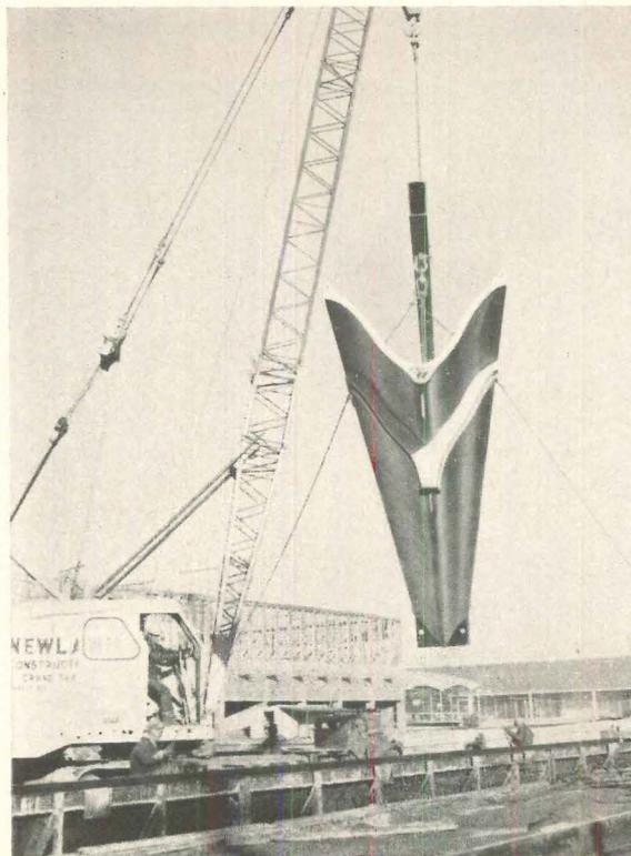
Prestressed concrete roof units were cast at the job site, using two casting beds. Prestress cables were placed first, followed by the cap form section. The concrete was form-cast by vibrating the lower form. The units were then covered with canvas and cured by using steam from college utility system. Roof utilizes 98 prestressed concrete elements with spans of 65 ft.
