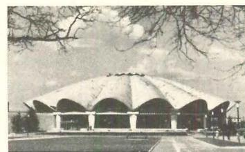
A tall, vaulted foyer leads into the 2,100-seat arena of the new State Circus in Bucharest (above and left). The roof is composed of 16 parabolas. Architects: N. Porumbescu, C. Rulea, S. Bercovici, N. Pruncu. Below, housing at Bucharest's Palace Square.
