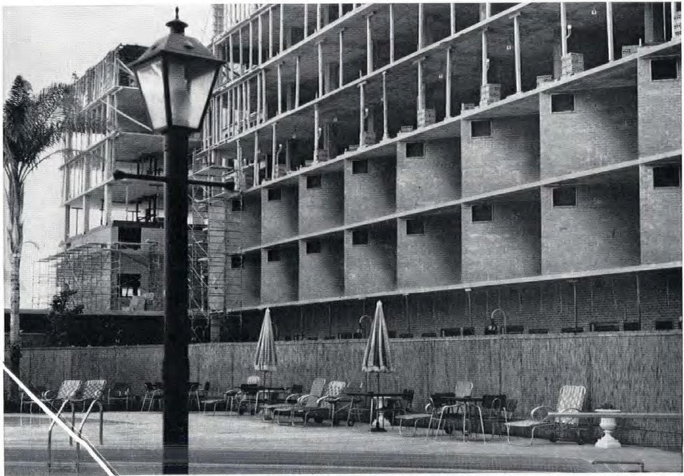
Installation is easy. Galvanized steel sleeves for General Electric Heat Pump Air Conditioning units are built in during construc-
