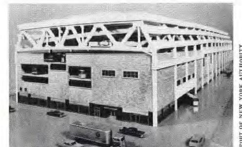
GIANT TRUSSES will support three new auto-parking decks over Port Authority bus terminal in New York without placing any additional load on remodeled structure below.
