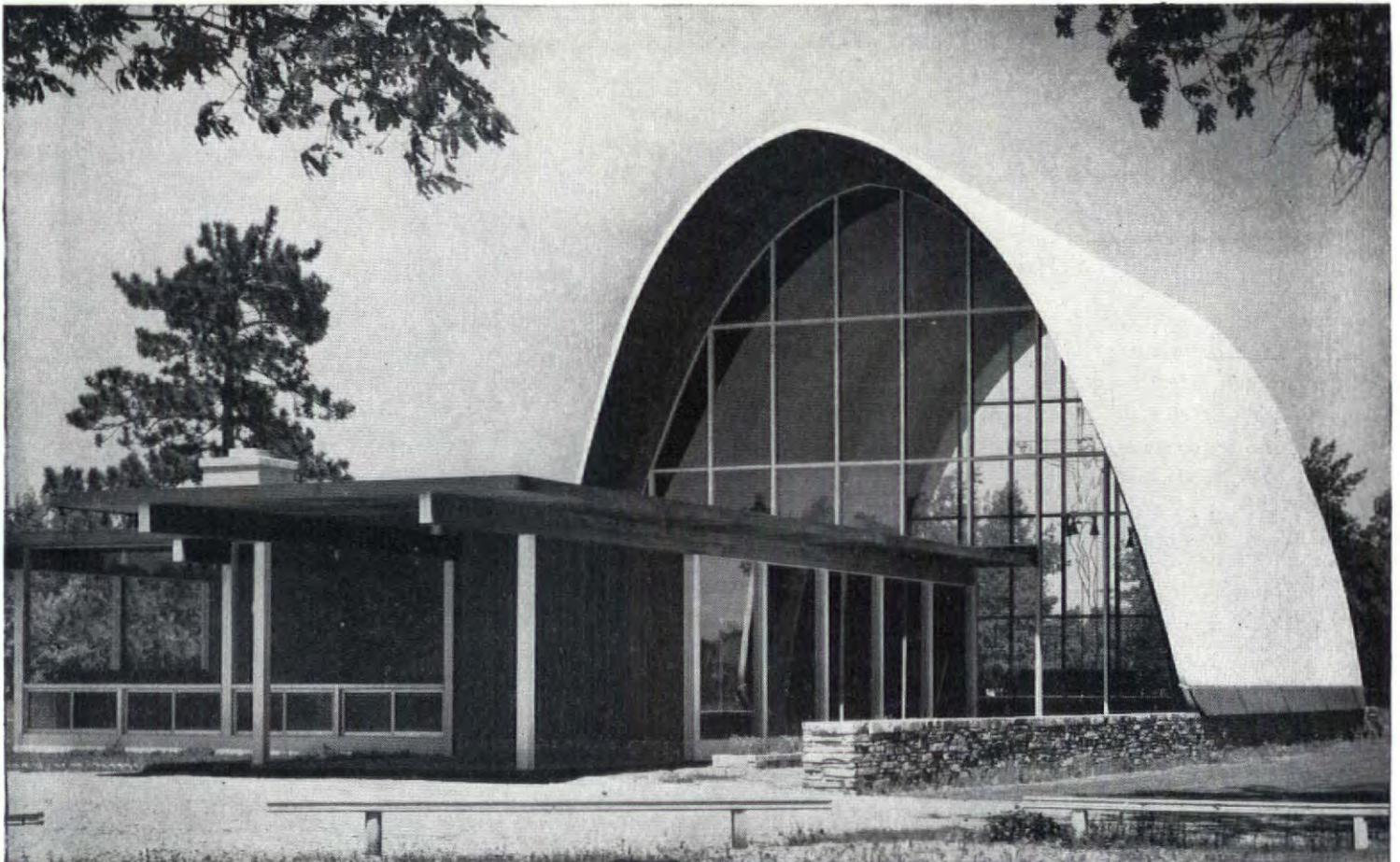
Gracefully bowed laminated beams supporting a parabolic arch, spacious wood-framed glass areas at either end—all combine to create a wide-open setting for a unique treatment of the crucifix. Note how simplicity of design dramatically demonstrates wood's quality throughout this unusual house of worship. Architect: Orus O. Eash.
