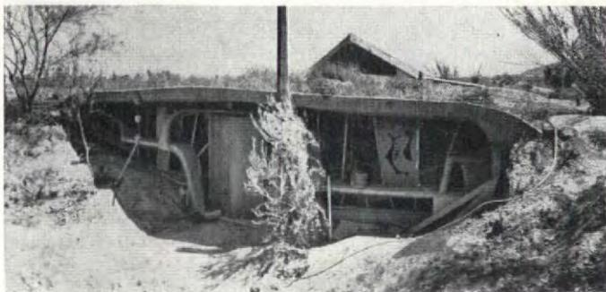
First "earth house" (above and right) is centered on a concrete fireplace sculptured to resemble a natural rock. Glass walls at each end of the house are interrupted by concrete stalagmites that serve as occasional shelves. Roof shell is being covered with planting.
