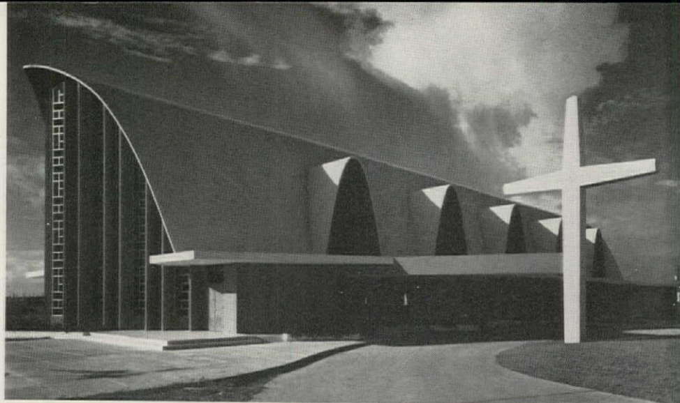
BARREL SHELL, graceful as the inverted hull of a ship, forms this church in San Juan, Puerto Rico, designed by O'Kelly & Mendez, engineered by Mario Salvadori of New York.
