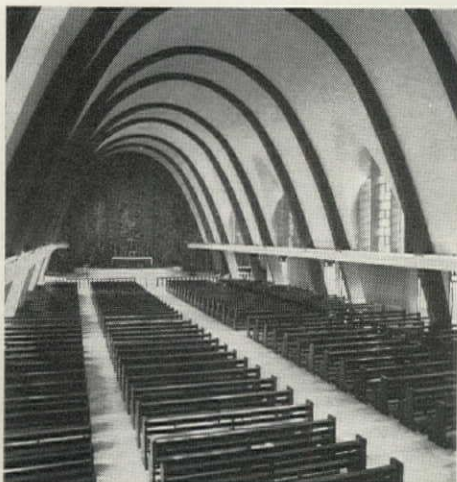
BARREL SHELL, graceful as the inverted hull of a ship, forms this church in San Juan, Puerto Rico, designed by O'Kelly & Mendez, engineered by Mario Salvadori of New York.
