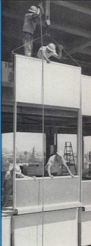
The lightweight (1.35 psf) grid units are installed from within the building, eliminating the need for scaffolding during erection. The factory-assembled units, stored at each floor level, are positioned individually and anchored to the building frame. Four men can easily handle installation of grid units.
