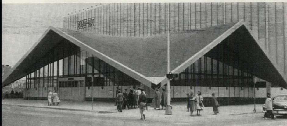
PARABOLIC CURVED entrance hall to May Co. department store in Denver, engineered by Roberts & Schaefer, is largest hyperbolic paraboloid shell in U.S.: 113 by 132 feet.
