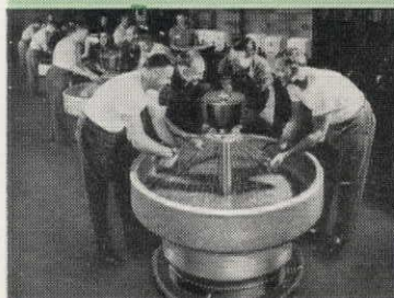
54-in. diam. full-circular precast stone Washfountains serve 8-10 simultaneously.
