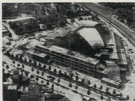
BIGGEST SHELL to be built thus far is rising in Paris on an incredible spiderweb of scaffolding and formwork. A triangular concrete shell roof, it will span a clear 720 feet to cover a huge Industrial Exposition Hall.
