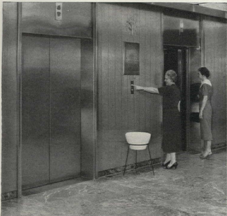
THE AMERICAN HARDWARE MUTUAL INSURANCE BUILDING in Minneapolis consists of two main elements: (1) a four-story office unit and penthouse; (2) a wing combining auditorium, employee dining facilities, and garage. Republic ENDURO® Stainless Steel is used for elevator doors, moldings, and fluted wall panels in lobby area. The softly finished metal enhances the beauty of the Monte Verde marble floor and Italian Cippolino marble walls. Yet, does not compete for attention.
