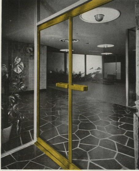
CURVED SECTION OF JAMBS and the stiles, rails, push bars and thresholds of exterior doors are bronze extrusions. (See detail below.)
