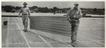
EASY TO PLACE. Galvanized corrugated Tufcor sheets arrive at the job site conveniently bundled and pre-cut to fit structural framing. No measuring or cutting is required. Three men can easily place and weld 5000 to 7500 sq. ft. of Tufcor in a single day. Low dead load of the finished Tufcor roof system (4 to 6 psf less than most types of roof construction) offers pronounced savings in the structural steel requirements.
