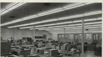
7. END-TO-END troffers attached to ceiling have main panels of Pattern No. 70 with Alba-Lite side elements. This arrangement provides optimum light and service conditions for new office in a large printing establishment.
