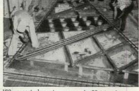
152 precast elements were used—80 triangles some perforated, others solid, and 72 solid quadrilateral panels-maximum sizes for panels 36 ft. x 10 ft.; for triangles 35 ft. on longest measure—maximum weights: for panels 10 tons; for triangles 5 tons.
