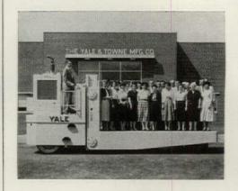
to only 1/20th the truck's 200,000 lb. capacity. The heavy-duty handler, in spite of its bulk and weight, is reported to steer easier than any passenger car equipped with power steering. Its 13' x 8' platform is designed to rise 2'4" hydraulically. Price: \$90,000.
