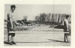
8' or will extend for a 4' cantilever without supplementary reinforcement. The system can be heavied up to meet ACI code requirements for a 100' live load over a 25' floor span in multistory buildings and, under normal roof loads, a 10" to 1' deep deck will stretch 30' or more. The two prefabricated components in the system—lattice trusses of 15 ga. cold rolled steel with cast concrete bottoms and masonry blocks—serve as forms for the concrete
