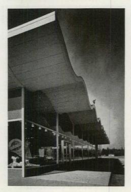
flat plates of light-gage steel, which rest on the lower flanges of the undulating steel beams. The entire roof is supported by two structural steel beams (not shown in photos) which stretch over the roof's 120' length, parallel to the wave crests, and rest upon four columns within the building. Thermal insulation boards are attached to the upper side of the ceiling, over which built-up roofing is applied.
