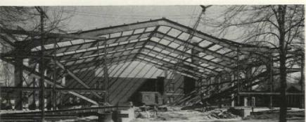
Approximately 240 tons of USS Structural Steel were used in the construction of the gymnasium. The steel framework was erected in seven weeks—joining accomplished by bolting and welding. The total structure—masonry, floor, seats, fixtures, everything—was completed and ready for use in 12 months.
