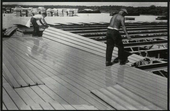
Easy installation of Milcor Steel Roof Deck helped save time in getting the Lincoln plant in Novi ready to produce 1958 models. The light-weight deck afforded additional savings on size and cost of structural members.
