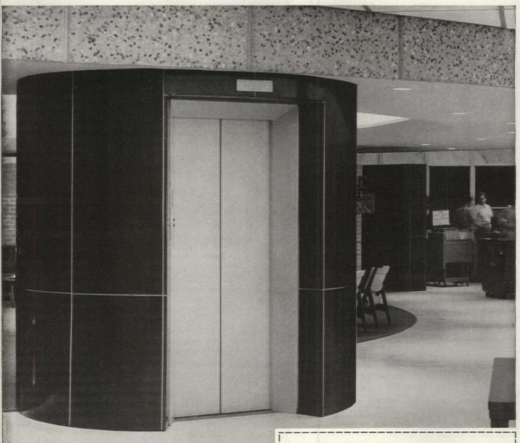
Unusual feature of the Charlotte, N. C., Public Library is this circular enclosure for the Rotary Oildraulic Passenger Elevator which serves four landings. The library is also equipped with two Rotary Oildraulic Freight Elevators.
