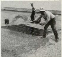
BUILT-UP ROOF. Rigidity and firmness of the Tufcor system provide a firm base for built-up roof, add years to the life of this roof, lower maintenance cost. Fast construc-
