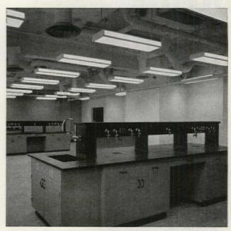
2. LABORATORY gets the kind of low surface brightness required for close work with these suspended troffers. Main panels are Pattern No. 70; sides of Alba-Lite provide excellent diffusion. Suspended troffers also permit fitting lighting fixtures around needed venting apparatus.
