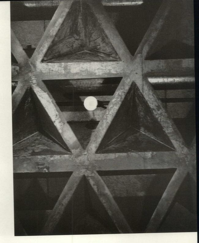
Yale Art Gallery and Design Center in New Haven used concrete without finishing. Imprint of the formwork remains evident, especially on the stair well (photo, left). The structure of the slab is a tetrahedral skeleton formed of T-beams, poured into re-usable forms. Oil from the forms mottled the concrete richly. Photographed straight up (right), this powerful slab also includes air ducts, electrical runs and acoustical treatment.
