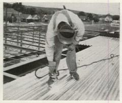
STRUCTURAL DECK. After tough-temper Tufcor sheets-80,000 psi and stronger-are welded in place, they help stiffen framing, provide an immediate work platform for trades. Tufcor easily withstands normal construction abuse.
