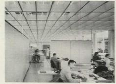
the metal-faced fins called for by the acoustical engineers, Smithcraft found itself in the perforated sheet-metal business. Another novel production problem was posed by the shape of the glass-fiber fillers. To make a double concave shape section that would not pick up inhibiting paint whenever the baffles were redecorated, a multiple-stitch sewing machine had to be found. Smithcraft men found two that could do the job—in a Boston antique shop.)
