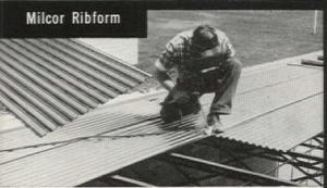
Rigid centering for concrete on spans up to five feet. Quickly installed — eliminates scaffolding — uses as much as 20% less concrete than flexible centering — permits monolithic finishing, without costly topping. For planning help, see Sweet's, Section 2F/In — or write for copy of Catalog 245.
