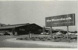
Supermarket (left) is the dominant building. Framed with steel bents, as is the rest of the center, it has a 90' span.
