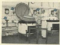
Ampoule Sterilizers regulated by Powers 252 Pressure Regulators and Valves.
