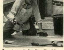
Easy to work. Installing Monel batten seam roof on a chapel of Washington Cathedral. Monel nickel-copper alloy is as easy to work as other roofing metals.
