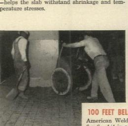
100 FEET BELOW, on the ground floor, more American Welded Wire Fabric is used. Style 6 x 6 - 4/4 in an eight-inch slab gives the floor strength to last and to stay attractive under heavy daily automobile traffic. Specify American Welded Wire Fabric Reinforcement for your concrete.
