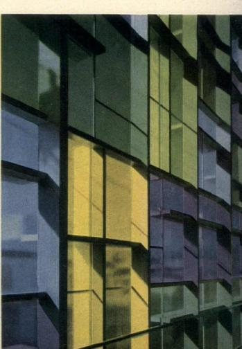
cast aluminum and buff porcelain enameled steel—create the interlacing pattern woven across the face of the Mile High Center's office tower. The buff-colored steel covers (and expresses) the underwindow air-conditioning units and their risers; the gray aluminum sheaths (and expresses) the building frame. To the right of the tower is the plaza and the curved roof of the transportation building; beyond them, the Center's remodeled bank building.
