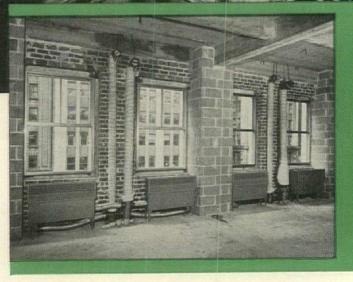
Photograph taken during construction of Seaman's Bank for Savings showing installation of Tuttle & Bailey Type MPW Double Duct Mixing Plenum Wall Units.
