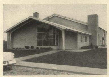
Low-cost office building shows striking modification with brick, glass and paneling. Large areas of glass are possible with no weakening of building, because entire weight is on Butler's rigid-frame.
