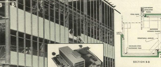
At left, Bel-Park Medical Building, Youngstown, Ohio, now under construction. Davidson Panels are assembled to window frames, then hoisted into place. Approximate time to install complete unit into building structure: two minutes. Architect, P. Arthur D'Orazio, Youngstown, Ohio. Contractor, Emanuel Katzman & Company, Youngstown, Ohio.
