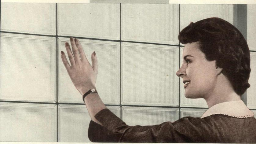
Solar heat input is greatly reduced. In a test during hot weather—when the outside temperature was  $90^{\circ}$ —the room side surface temperature was 14 degrees less than that of a conventional type light-directing glass block.
