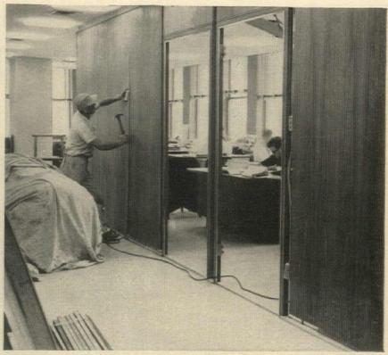
PARTITIONS ARE INSTALLED without costly interruption of regular office routine. Workman is shown installing section of Weldwood Movable Partition; completed corridor is shown at left.
