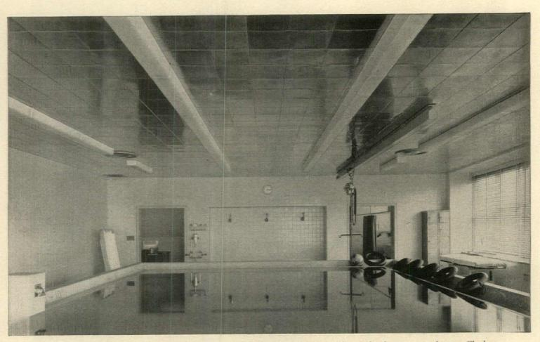
Moisture can't damage the Armstrong Arrestone ceiling in this therapeutic pool room. The bare mill finish of the aluminum pan is rustproof, and moisture has no harmful effect on the mineral wool pad backing. Arrestone is also easy to clean. It's incombustible, too.
