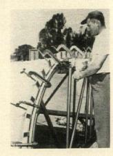
ate, the Californian swimming pool manufacturer is making the 10,000 gal. pool in four matched shell sections. Designed for either oven curing or cold layup fabrication with self-curing resins, and weighing under 900 lb., the four pool sections can continued on p. 224
