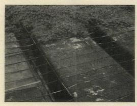
PAN AND SLAB construction was used for the roof of the garage. Three inches of reinforced concrete were poured over 10-inch-deep pans. American Welded Wire Fabric—style 6 x 12 - 5/5—helps the slab withstand shrinkage and temperature stresses.
