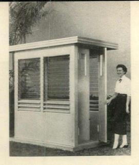
rigid honeycomb core prevents any surface deflection or waviness in the metal facings. Selling for about \$1.50 to \$3.00 per sq. ft., the panels and doors may be ordered with smooth or embossed aluminum facings in an anodized finish, or prepared for paint coat. Wall panels also are obtainable with porcelain enameled skins. Doors are available in sliding, pivot and fold-up styles. Insulation value of a 3" thick Panelfab
