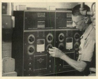
Dunham VARI-VAC Controls in Quality Hill Towers provide centralized, one-man operating station for all adjustments, settings and remote control readings for 100 apartments.
