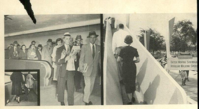
Here's the world's first commercially successful SPEEDWALK in operation at an eastern railroad terminal. In less than two years it has handled almost 2 million passengers. By eliminating a fatiguing uphill climb the moving sidewalk has increased commuter travel 4½%, countering a downward trend in revenue.
