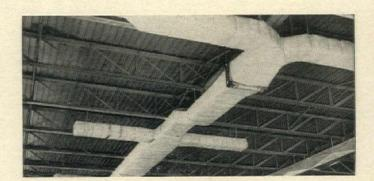
A large section of heating and cooling ducts insulated with L·O·F Super Fine. Ducts were coated with adhesive, then wrapped around with Super Fine and secured with light-gauge
