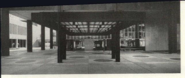
Entrance canopy is a free-standing structure of black-painted steel, roofed with 30 glass-block toplights each 3'-2½" x 6'-2". Fixtures under cross members bathe entrance in a pool of light at night. Seen through arcade at left is remodeled building which forms one side of lower plaza.
