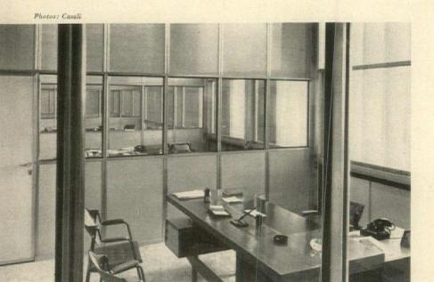
Interior partitioning, all demountable, is made of aluminum sheets, connected to each other and to ceiling with rubber joints, under pressure. These partitions are of three types: opaque panel, glass panel in center; glass panel near ceiling. Special study was made of acoustical problems. Decibel losses were figured at standard room noise level of 70 db., for three partition types are, respectively, 18 db. absorption, 20 db. and 18 db.
