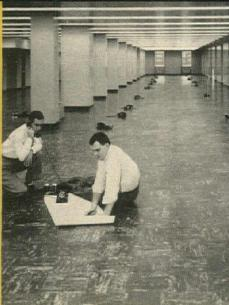
Connecting some of the 1500 telephone outlets installed in the R/C Duct Floors.
