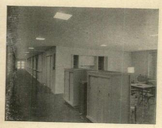
By muffling noise of footsteps and voices, the Cushiontone ceiling keeps this corridor and adjoining TV area comfortably quiet. Cushiontone's white paint finish can be cleaned or repainted easily without loss of acoustical efficiency.
