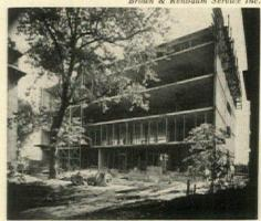
SLAB EDGES ARE CAMBERED upward until set to allow for curing deflections.
