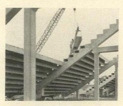
channels spaced 32' o.c. on a reinforced concrete frame, were only \$13.50 per bleacher seat (not including utilities or preparation of playing field). Since that structure was built, slight modifications have been made in the channel design to make it serve as a complete bleacher seat,
