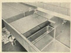
POT SCULLERY — Close-up of round-corner stainless steel pot and pan sink. Compartments, drainboard and back splash form one continuous crevice-free surface, simplifying cleaning. The sliding tray permits placing of pots at convenient work height.
