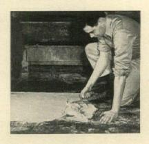
job and handled like regular concrete or mortar. It may be troweled or buffed to a smooth finish. Its rubber content makes the cured composition so flexible that a long thin strip can be bent by hand into a hoop. The surfacing's special cement gives it excellent bonding to almost any clean hard surface: Laticrete's grip on masonry is 300 lb. psi. It will also adhere to metal, and to glass for a pull of 100 lb. psi.
