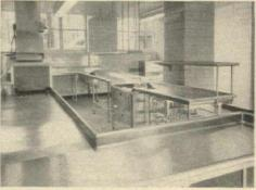
STAINLESS STEEL DISH TABLES in dish pantry. Work top and raised rolled edges form a continuous, crevice-free surface to assure maximum cleanliness.
