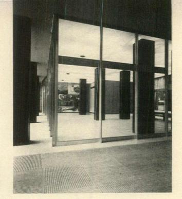
**Exhibition space** on first floor is flooded with light from egg-crate ceiling. Columns are sheathed in black and white anodized aluminum.
