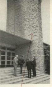
Brick is local product with pinkish cast and together with integrally colored buff mortar looks very handsome, has needed no pointing. Only two defects are observable in school's condition: 1) efflorescence has appeared on front portion of chimney-clocktower where it is neither sheltered by eaves nor warmed by flues, 2) hedges need a haircut.
