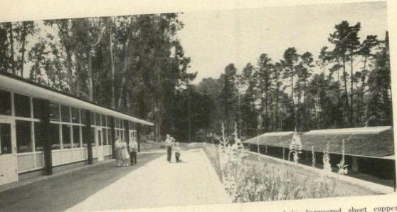
Upper wing: exterior columns are steel sections, encased in lacquered sheet copper
