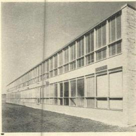
Neill Junior High School, North Chicago, Illinois. Featured are the Alumiline special design Curtain Wall members, along with 5" tubing around the door frames only. The wall shown is approximately 22' high by 188' long, with an identical wall on the opposite side of the building. Fabricated and installed from Alumiline sections by The National Glass Corp., Chicago, III.
