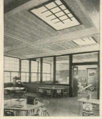
The combination of light-directing glass block and vision strip keep brightness at comfortable levels, provide vision and ventilation.
