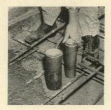
closure. The other metal end is then inserted in the top of the sleeve and anchored to the form to hold it straight. After the concrete sets, closures are knocked out leaving a neat opening for pipe or conduit. Where sound insulation is important, the sleeve itself can be left in. Sonopipe in the 4" size runs about 18¢ per ft., FOB factory, and metal ends to fit that size are 6¢ apiece.
