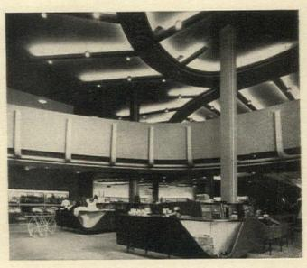
Kline's West, Carrier-equipped department store in St. Louis, has a unique air duct system. Conditioned air comes from "trees"—ceiling-suspended, tree-like lighting troughs centrally located over main floor and mezzanine.
