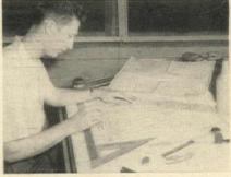
New design is added to the Autopositive, which has dense photographic black lines on a clean white translucent base. Required number of shop prints—each crisp and uniform—are produced from this master, which can also be used later on for minor revisions.
