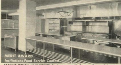
COOKING SECTION, MAIN KITCHEN: Food conveyor traffic flows rapidly around this section in a counter-clockwise direction. Ample work surfaces are provided by the generously-proportioned cooks' tables. Note seamless work tops, rounded corners, welded tubular undershelves.
