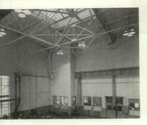
MERCURY LAMPS, in groups of three 1,000-w. units, provide 50 foot-candles in hangar; small incandescent lamps provide standby lighting.
