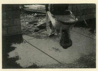
QUICK, EASY INSTALLATION . . . Premoulded Membrane is a strong, permanent vapor seal that will resist the trundling of wheelbarrows and the impact of aggregate during the pouring operation . . . best of all, with Premoulded Membrane you don't need an expensive underlayment of sand to absorb shock. This strength to resist tearing and puncturing is very important . . . as a vapor seal is much like a child's balloon, for only a small hole renders it useless.
