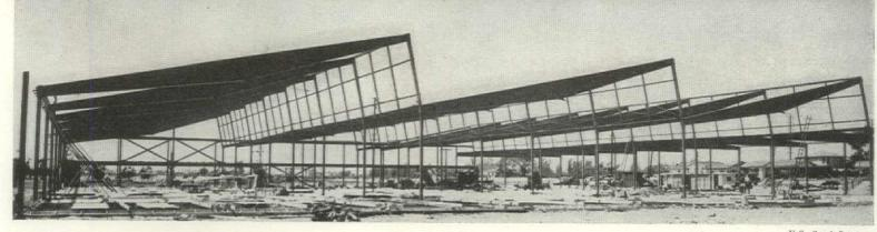
TAPERED GIRDERS 60' long were built up from steel plate for factory (above). Alternate method (sketched at right) is to flame-cut web diagonally, turn pieces end-for-end and butt-weld them together.
