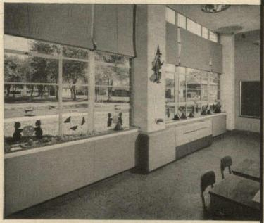
MICHIGAN. Installation of Herman Nelson Unit Ventilators at the Ralph J. Bunche School, Ecorse, Mich., features unique DRAFT|STOP Wall which, in addition to eliminating window downdrafts, serves as an economical wall finish. Note how filler section fits around pilaster—another example of Herman Nelson flexibility. Superintendent of Schools: Ralph E. Brant; Architect: Bennett & Straight; Engineer: Benjamin Schulz & Associates; Mechanical Contractor: Standard Plumbing & Heating.
