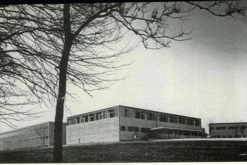
Highway view of office trio corresponds with work-flow diagram (below). Working with layout and building shapes predetermined by office efficiency studies meant added sitework to keep floors at equal levels, resulted in identical building heights and problems of distribution and storage.
