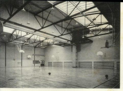
**Gymnasium** is framed with bowstring trusses on steel columns. Divided, each side gets skylight. Rolling bleacher storage can be seen along wall. Girls' lockers are at floor level, boys' at lower level.
