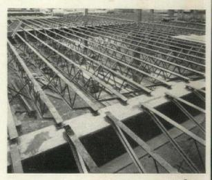
Pittsburgh's new Grant Store is built with Truscon "O-T"® Steel Joists. Open Truss Steel Joists are lightweight, fire-resistant, rigid and economical. They provide low-cost-per-square-foot construction with adequate strength and safety. They are self-sustaining. Any number of floors can be erected at one time with joists serving as working platforms. NOW! TRUSCON offers a NEW CLERESPAN® STEEL JOIST 96 FEET LONG. Write for details.
