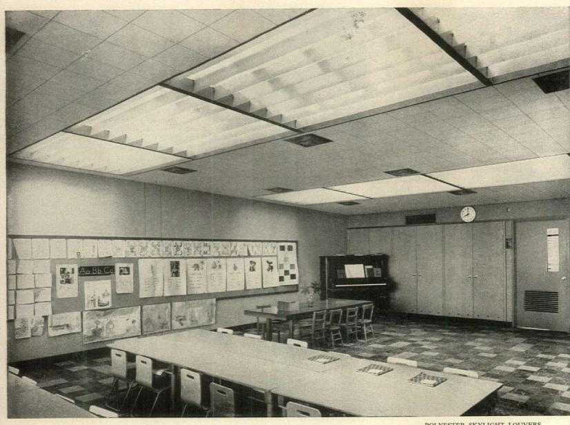
POLYESTER SKYLIGHT LOUVERS provide soft, diffused light, and have specific flame spread rating that meets code requirements in most areas.
