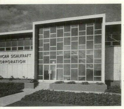
Entry stairwell projects from row of offices, is glazed in frosted blue and clear amber panels, set off by brick-red base. Siding is corrugated asbestos board.
