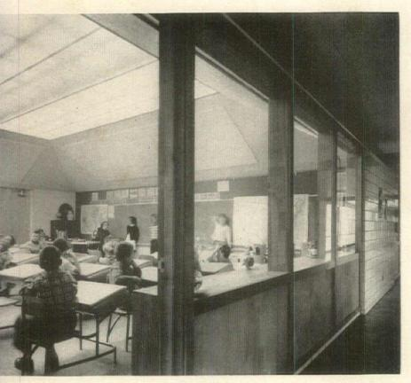
**Skylights:** above, at Grosse Pointe and, below, for two of Architect Yamasaki's most recent school jobs. In this simplification, skylight bar holds both glass and ceiling.
