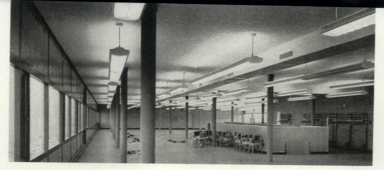
Open offices in Service Co. and RCA Victor buildings are divided with minimum of low partitions. Acoustical tile, ducts, lights are attached directly to underside of slab. Above and below vision strip are low-maintenance panels of porcelain enamel.
