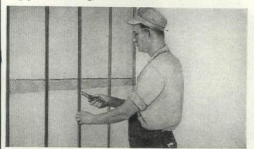
**6.** 2" SOLID PARTITIONS, METAL BASE SYSTEM — easiest, most economical solid plaster partition possible. Here, Wheeling Bantam Diamond Lath is attached to Channels with Wheeling Hank Tie Wire.
