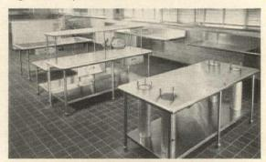
SALAD AND VEGETABLE PREPARATION UNIT — View shows convenient position of work tables in relation to sinks. Note how ample spacing between units permits freedom of movement for personnel. These layout factors help speed procedures. Wall-mounting of stainless steel sinks in background eliminates leg obstructions, permits thorough cleaning of floor surfaces.
