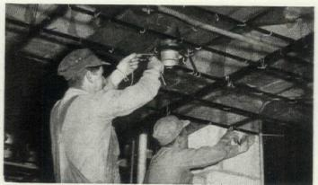
3. SUSPENDED CEILINGS – permits complete design flexibility plus multiple practical applications. Wheeling Channels, Metal Lath and plaster can be shaped to meet the most complex conformations.
