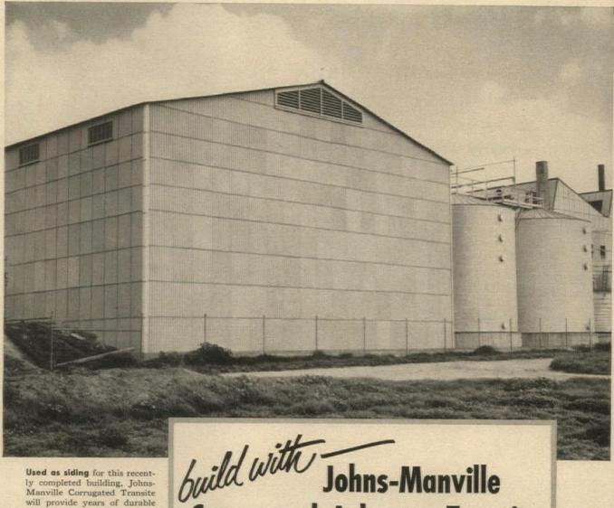
Used as siding for this recently completed building, Johns-Manville Corrugated Transite will provide years of durable service and fire safety with a minimum of care. It needs no paint or special treatment to preserve it.
