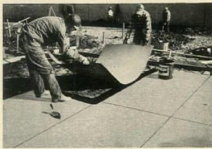
IDEAL FOR ALL CONSTRUCTION APPLICATIONS... Premoulded Membrane, supplied in 4' x 8' sheets, is laid directly over the hard tamped\* grade with a 6" overlap. This overlap is then sealed with Sealtight Catalytic (non-setting) Bonding Asphalt—giving you a monolithic vapor seal that will expand and contract with the slab above ... without breaking the seal. You actually form a vapor proof "saucer" into which the concrete is poured.
