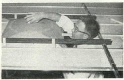
or besmudged tiles may be replaced individually without disturbing anything else in the ceiling. When new tenants take over office space, troffers can be relocated easily. The entire ceiling is in fact demountable and completely salvageable. In-place cost with top-grade acoustical tile is estimated at 70 to 80¢ per sq. ft. depending on size of job and local labor.
