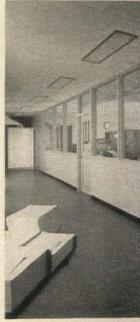
Ceco Hollow-Metal Doors are used throughout the building, in borrowed-light partitions and in separate openings, as shown in these two pictures.
