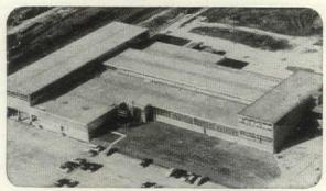
Eighty thousand pounds of Alcoa Aluminum was used in the seventy-five thousand square feet of Fenestra Panels completely shop-fabricated for the Airport Terminal. Detroit Steel Products Company's Pittsburgh plant is enclosed with similar panels.
