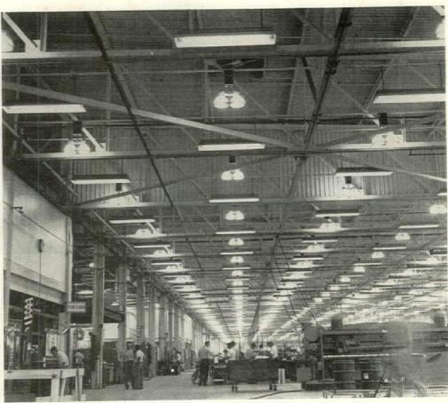
DUAL LIGHTING: 400 w. mercury and 85 w. fluorescent lamps provide 100 foot-candles in Rohr Aircraft plant in Riverside, Calif.
