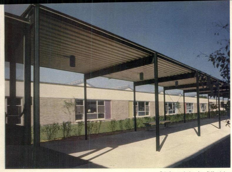
**Exterior** emphasizes low 7'-2" window-height line; brick above was sprayed with concrete. Brick and white stripes, with panel accents of color, produce effect charmingly and surprisingly "miniature."
