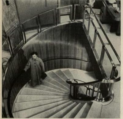
THIS CIRCULAR STAIRWAY leads from the banking floor to the vault room in the first basement floor. Stainless Steel handrails curve on changing radii to accent graceful curve of stair. Guard rail at top consists of stainless frames with glass screens to preserve appearance of openness and space.
