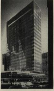
Lever House (above, plan below) has services at end, 6,000 sq. ft. with inside columns and stair.
