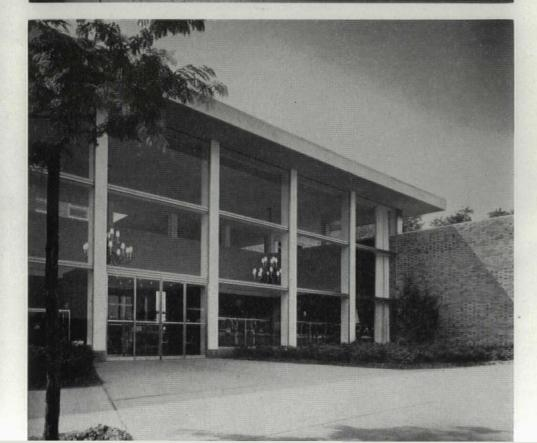
Exterior of main entrance shows how building is handsomely textured in varying shades of gray glazed brick (with magnesium-spot or "salt and pepper" pattern), trimmed in white Vermont marble and stainless steel. Building provides 70,725 gross sq. ft. of floor area, cost about \$21 per sq. ft.
