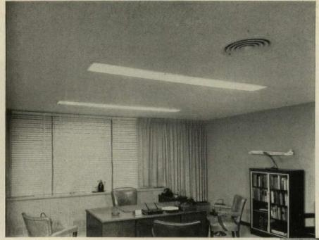
The high acoustical efficiency of this Travertone ceiling provides the undisturbed quiet needed for concentration. Travertone is quickly installed by cementing or suspension methods and can be scored and cut to fit around fixtures.
