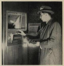
"HOLD-UP PROOF" is this after-hours banking "snorkel." This is the view from the customer side. There is an elevating device, periscope and telephone connection. All bright metal is stainless steel.
