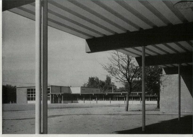
Covered play space at south end of school has steel columns. Otherwise, prestressed columns, prestressed beams and steel deck are used. Leader hugs foreground column.
