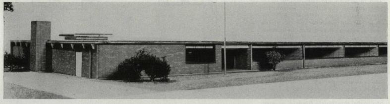
School model has wall of glass, made possible by elimination of structural piers.
