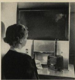
AFTER BANKING HOURS, this "snorkel" permits the teller, safely seated in the basement vault room, to receive payments or deposits from customers outside of the bank. Stainless Steel is used for the work surface, as well as all other metal parts.
