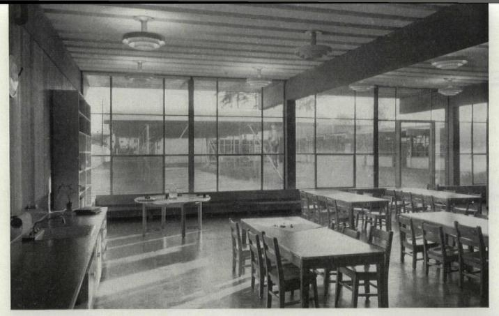
Classrooms are two bays wide, 28'-8" x 33'-10". View above shows kindergarten, looking end-on at arched play shed. Photo at right shows typical classroom at corridor wall and partition. Prestressed beams were cast in steel forms using 10,000 psi compressive strength, no-slump concrete. To vibrate
