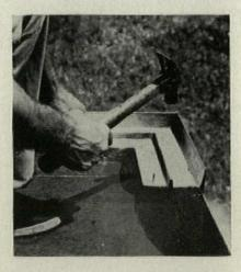
corners are stock items, and all G-S units are made in copper as well as steel. In installation, the sections may be overlapped 2" and bedded in mastic. Grooved wood driving blocks are provided for pressing sections into a good mechanical bond. As an alternate technique, joints can be butted and soldered. G-S Gutter extends 3" over the fascia; it may be painted or left as is.
