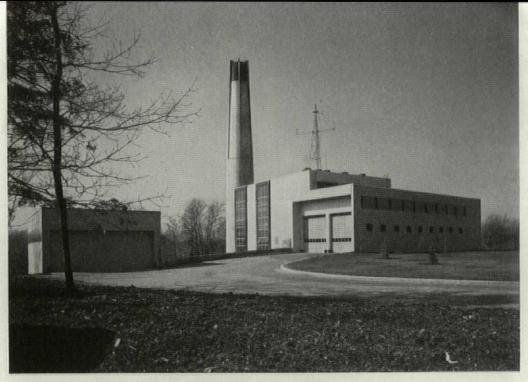
Truck entrance is on upper level so that dumping process in aided by gravity.
