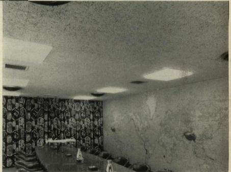
Completely incombustible, Travertone meets all fire-safety regulations. Its handsomely fissured surface resembles travertine marble and can be washed or repainted as often as desired without impairing its acoustical effectiveness.
