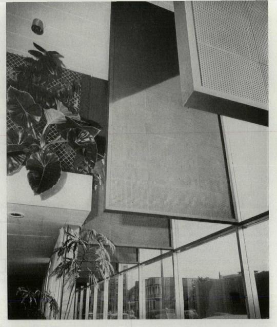
Inside fins, 5' apart, are attached to structural aluminum mullions of blue glass wall.
