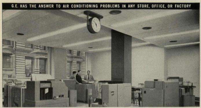
Acoustical hung ceiling holds supply ducts and registers for distributing air cooled by G-E packaged units. Furred space itself acts as plenum for return air, entirely eliminating need for second set of ducts.
