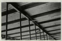
supports would be necessary only at the ends and middle of the pan forms.)
