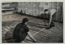
HEAT FOR THIS basement game room will be provided by ½" PG's embedded in concrete. For floor or ceiling installations the pre-formed Anaconda Panel Grid offers many economies.
