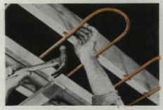
PG's ARE EASILY INSTALLED—A %" PG weighs only 10 pounds, is easily lifted and propped in place, leaving worker's hands free to fasten straps. Here, metal lath goes under the PG's.
