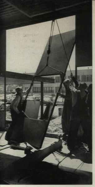
INTEGRATED WALL FRAME being installed at Midway Airport, Chicago, is prefabricated complete with sash and insulated porcelain enamel panel, costs \$3 per sq. ft. erected.
