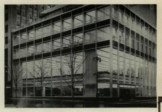
A Engineering complication in the construction of the new Manufacturers Trust Company Office in New York dictated the need for an unusual cantilever application. Girders, 70 feet long and weighing seven tons each, stretch in two directions from the supporting columns, which are set back from the building line. The 43rd Street cantilever extends 20 feet 5 inches from the column line. Only eight exposed columns are on the main banking floor—an area of 11,000 square feet.
