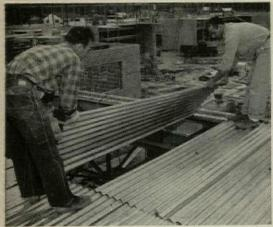
Quickly Placed. Tufcor and Corruform sheets are delivered to job site pre-cut to fit framing. A crew of two or three men can easily place 5,000 to 10,000 square feet, in a single working day.
