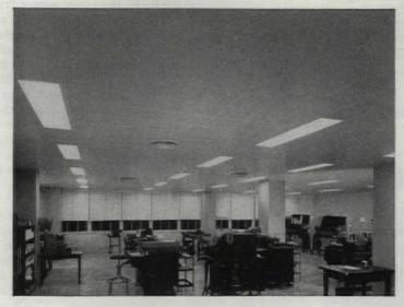
Sound conditioning this punchboard accounting machine room required an efficient acoustical material. Armstrong Arrestone was chosen for its high noiseabsorbing qualities as well as its easy maintenance.
