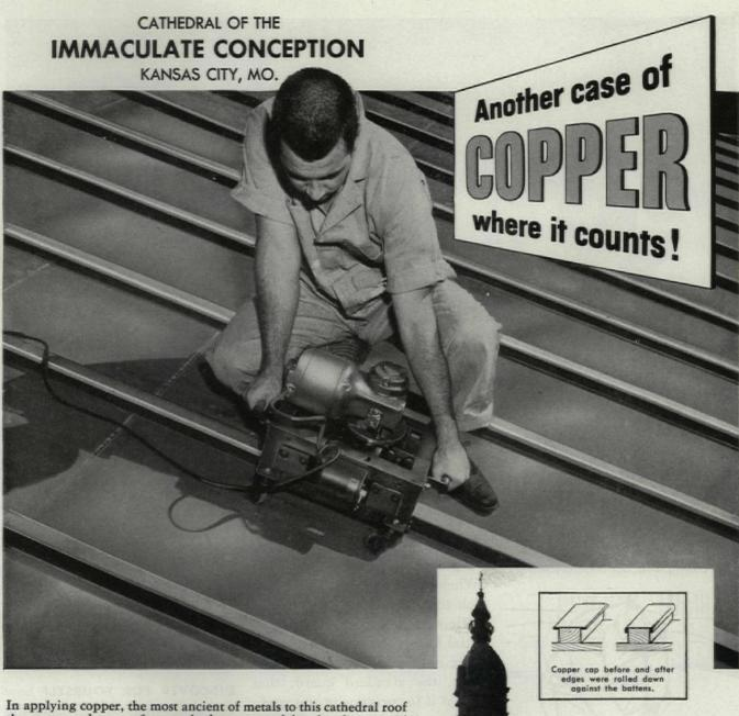
In applying copper, the most ancient of metals to this cathedral roof the most modern roofing methods were used by the sheet metal contractor, A. Zahner & Company. The machine you see above was developed by this Company to form the last fold of the copper cap over the battens. Not only does it do the forming more neatly but, according to the contractor, it does this job 10 times faster than would be possible with hand tools!
