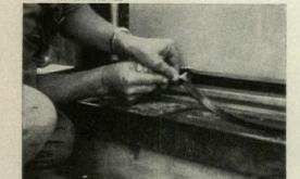
GM has used porcelain enameled panels since 1951, when it put one of the first enameled curtain walls on its administration building (AF, Nov. '51). The latest panels average 3'-6" x 4'-6" (maximum 4' x 9'-6") and are set in 3'-9" wide extruded aluminum frames.
