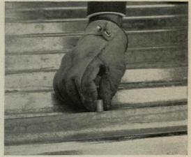
Vent Clip Prevents Vapor Pressure Build-up. Granco vent clips, inserted on lip of each sheet, one between each support, prevent vapor buildup in roof slab under intense summer sun.
