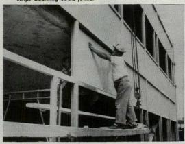
"Our unique panels combine ultra-modern appearance and high insulating efficiency (U factor 0.15)... cost just \$4.50 per sq. ft. erected in place.
