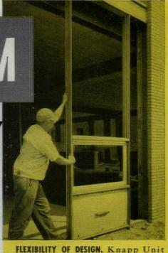
FLEXIBILITY OF DESIGN. Knapp Unit Wall Panels are assembled at the factory with the exception of glass. Each unit is complete with insulated metal panels and ventilator com-pletely caulked. They provide full flexibility of design. Ventilators, fixed glass and insulated panels can be varied to meet the individual requirements of the job.
