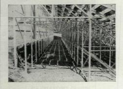
All Snyder grandstands and bleachers, with the exception of seatboards and footboards, are built throughout of structural steel, making Snyder Steel Stands Safer.
