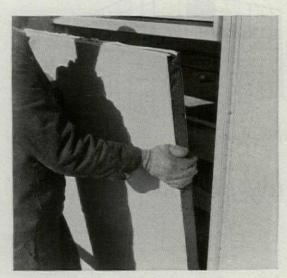
on this school building. Note the inorganic insula-tion between face and inside sheet. Edges of panels are carefully grouted to make wall water-tight.
