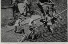
SNOW MELTING SYSTEMS are installed easier and quicker with ½" PG's embedded in concrete.
