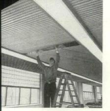
Easy access to ceiling. A can lift any one of the lightweight sections and slip it over an adjoining strip to get to area above.
