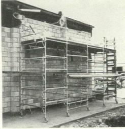
tower in just 8 minutes. Each framing unit is load tested at 400 lbs. psf. The standar-dization of parts also helps keep the price within reason. Framing for a structure 35' long, 20' high and 5' wide would cost around \$600, or about 87¢ per sq. ft.
