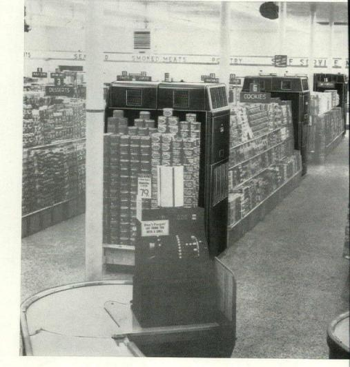
Six 5-ton Frigidaire Self-Contained Air Conditioners are installed in pairs, back to back. Note four-way air distribution without ducts or special grilles.
