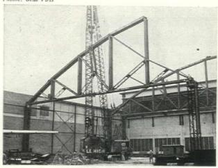
Projecting trusses rise 25' above roof of Fairchild factory extension to span 200'. At top of photo prefabricated sections are being assembled.
