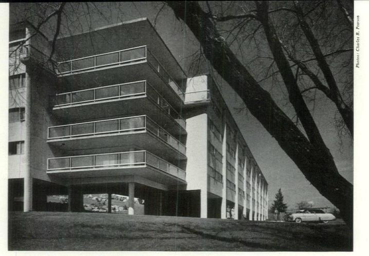
Wing intersection saves stairways and creates an opportunity for wide double-exposed porches on each floor. Open first floor minimizes drainage problems. Note exterior framing, another money-saving design element.
