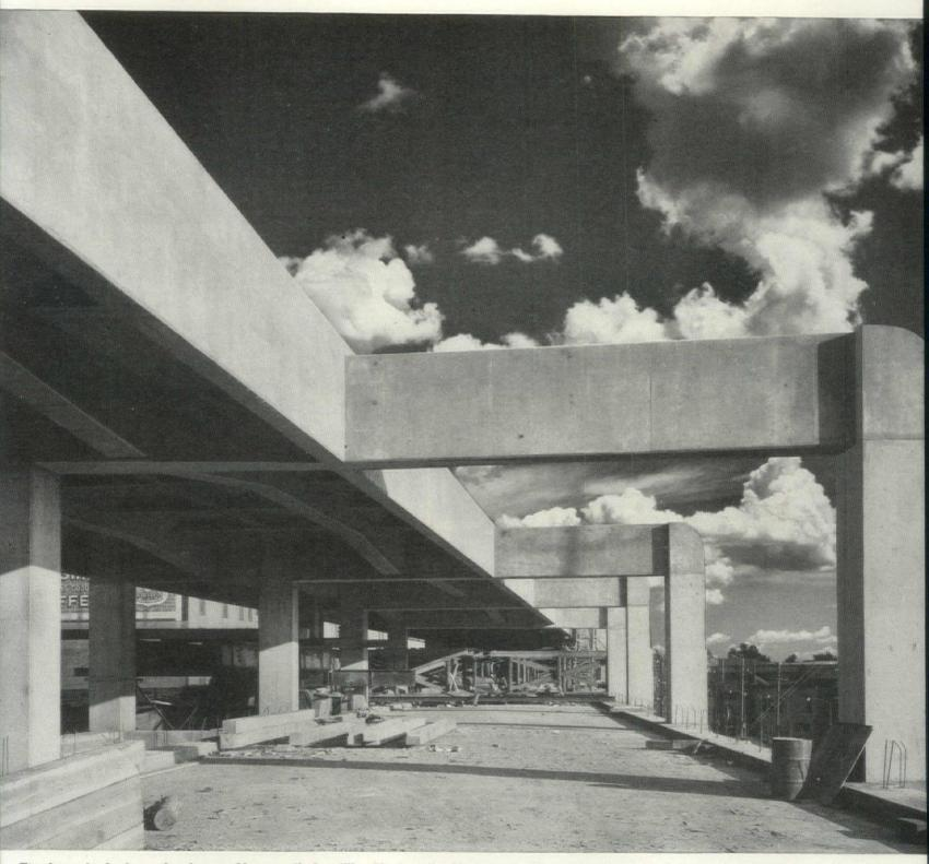
Fir plywood solved complex form problem on Alaskan Way Viaduct. Double-decked structure .77 miles long required only 400,000 square feet of plywood.
