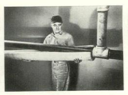
nolic resins, is factory-formed into resilient cylinders. It has a very low K factor—.23 at 100° mean temperature—and is extremely light and easy to handle. Each 6′ long section is spread apart at the slash, slipped over one end of the pipe and snapped into place. The seam is then closed with tape, staples, string
