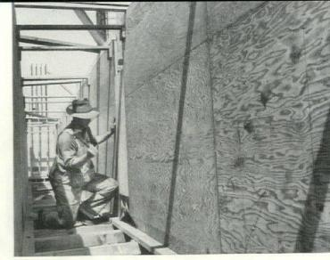
Beam and girder bottom forms were built up inside standard vertical form panels in what contractor called "floating beam bottoms." System simplified handling of variable beam and girder depths.
