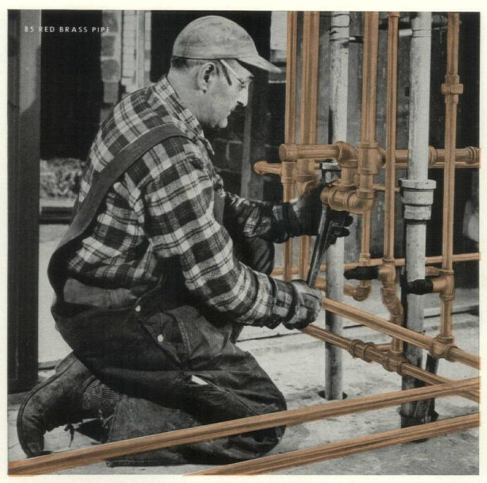
BACK TO BACK, two second-floor bathrooms, for semi-private rooms. AnacondA 85 Red Brass Pipe for hot and cold water lines.
