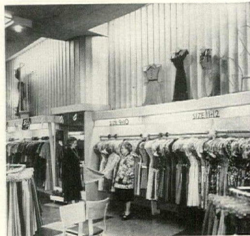
KAISER ALUMINUM SIDING, installed vertically in The Cotton Shop, Chicago, gives effect of height, fits curved surface, hides heavy columns. Baked-on enamel coat is smooth, easy to clean, lasts longer. Architects: Walter H. Sobel, J. Stewart Stein. Contractor: Lee Construction Co., Chicago.
