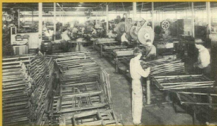
Ventilating portions of the windows are assembled first, by air hammer riveting and automatic flash welding.
