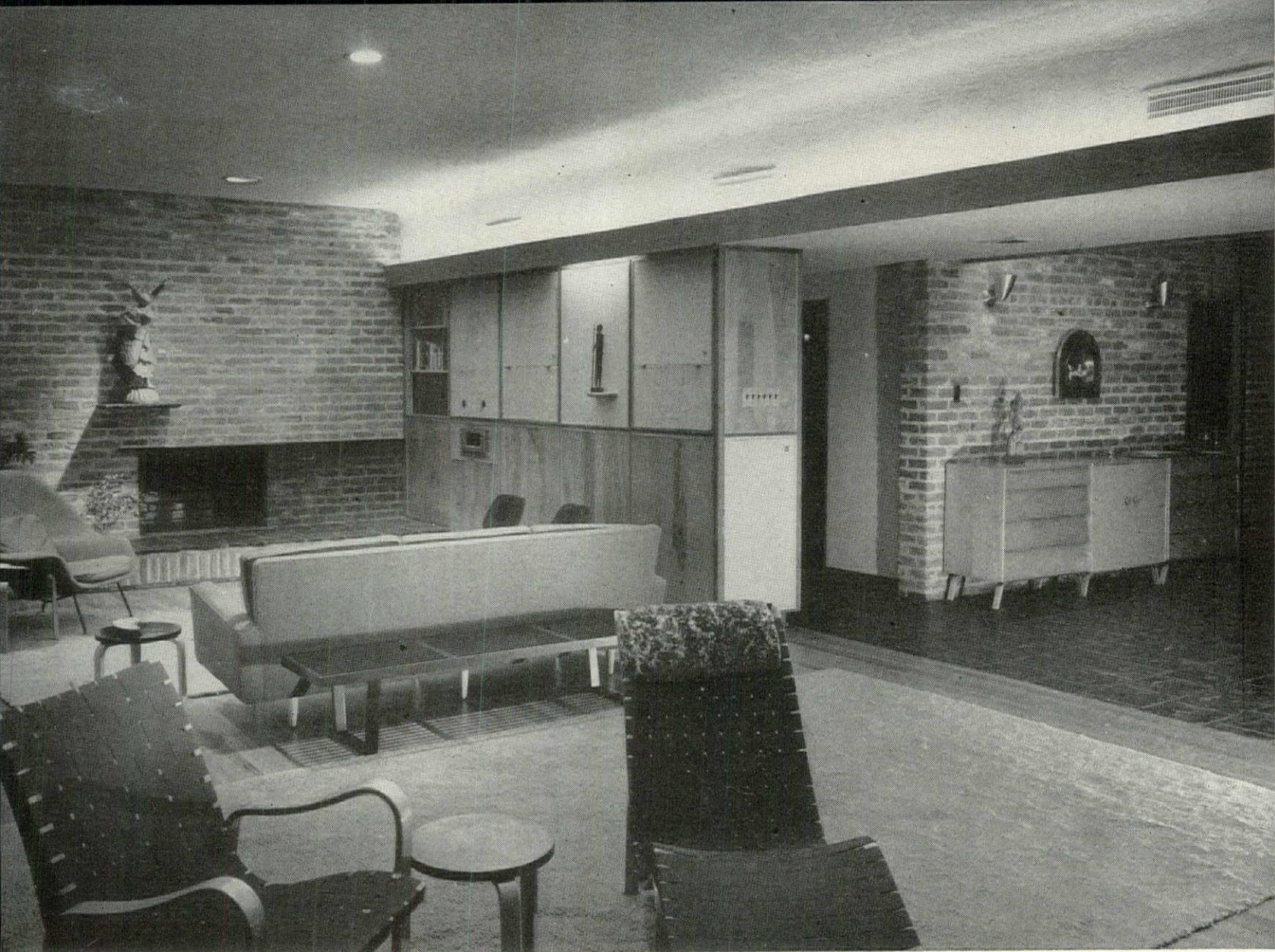
Overhang (foreground) provides additional route to rear. Patio permits outdoor dining in full privacy. House combines air conditioning ducts with indirect lighting (photo below). Fluorescent tubes are recessed on living and dining room sides of furred-down ceiling, direct hall spots are inset flush with duct itself.
