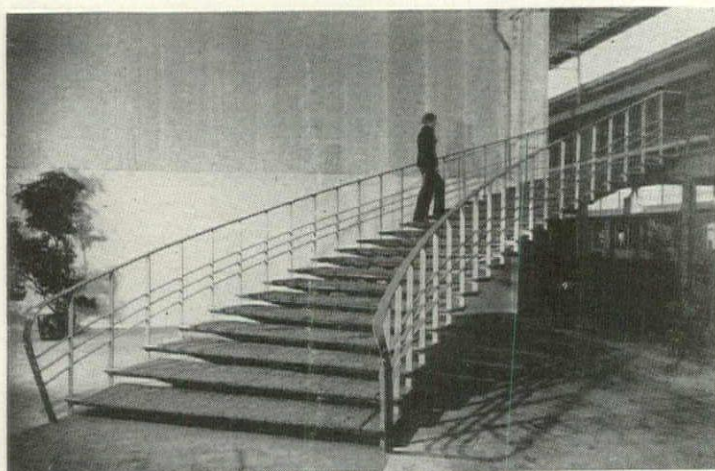
HANNOVER: Also part of "Constructa" exhibition was this cantilevered, steel spiral staircase shown by a stair manufacturer.
