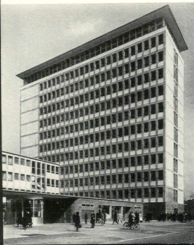
FRANKFURT/MAIN: 12-story office tower for A.E.G. electrical concern is located near Frankfurt's new "Bridge of Peace," was designed by Architect Assmann
