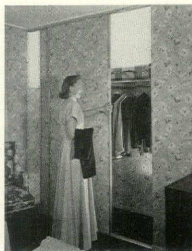
Sliding doors of pressed fibre board in 1950-51 house made closet construction cheaper, opened bedroom to living room.
