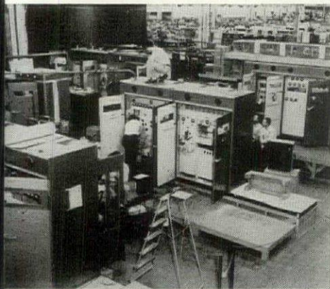
New warehouse space will be added at Electronics Park as shown in air view below. Television picture tubes made in tube building will be carried to warehouse in back of receiver building by a long out-of-doors conveyor. Transmitter building needed its own warehouse because of last-minute testing of equipment as shown in photo (L.).
