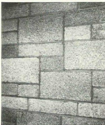
Close-up showing sizes, texture and joint treatment.
