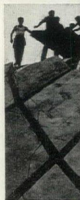
The web of strips visible in the ceiling does not support the cupola. That job is done by curved diamond shaped slabs which rest between and above the ribs (which are only separators and stiffeners).
