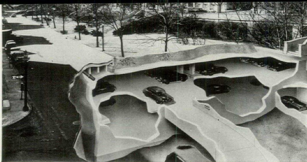
BALTIMORE'S PROPOSED UNDERGROUND GARAGE, while potentially helpful to reduce downtown parking problem, also is urged by city leaders as an air raid shelter despite objections of civil defense experts. Each level would contain four rows of 100 cars each.
