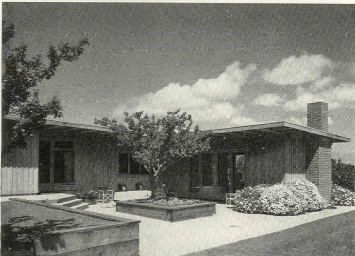
Wurster, Bernardi & Emmons did this house several years ago in California. While this is considerably larger than a typical builder's house, it shows the value of an L-shaped design with a wide overhang (plus landscaping) for a house with a flat roof.
