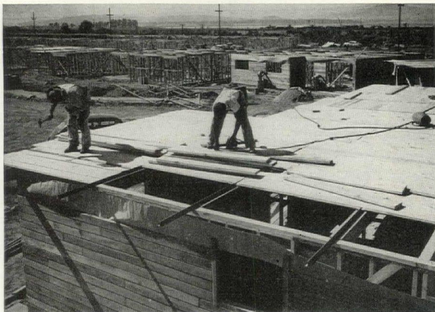
Above: carpenters installing planks on one of Smith's flat roofs. Note steel T-bars for cantilevering overhangs.
