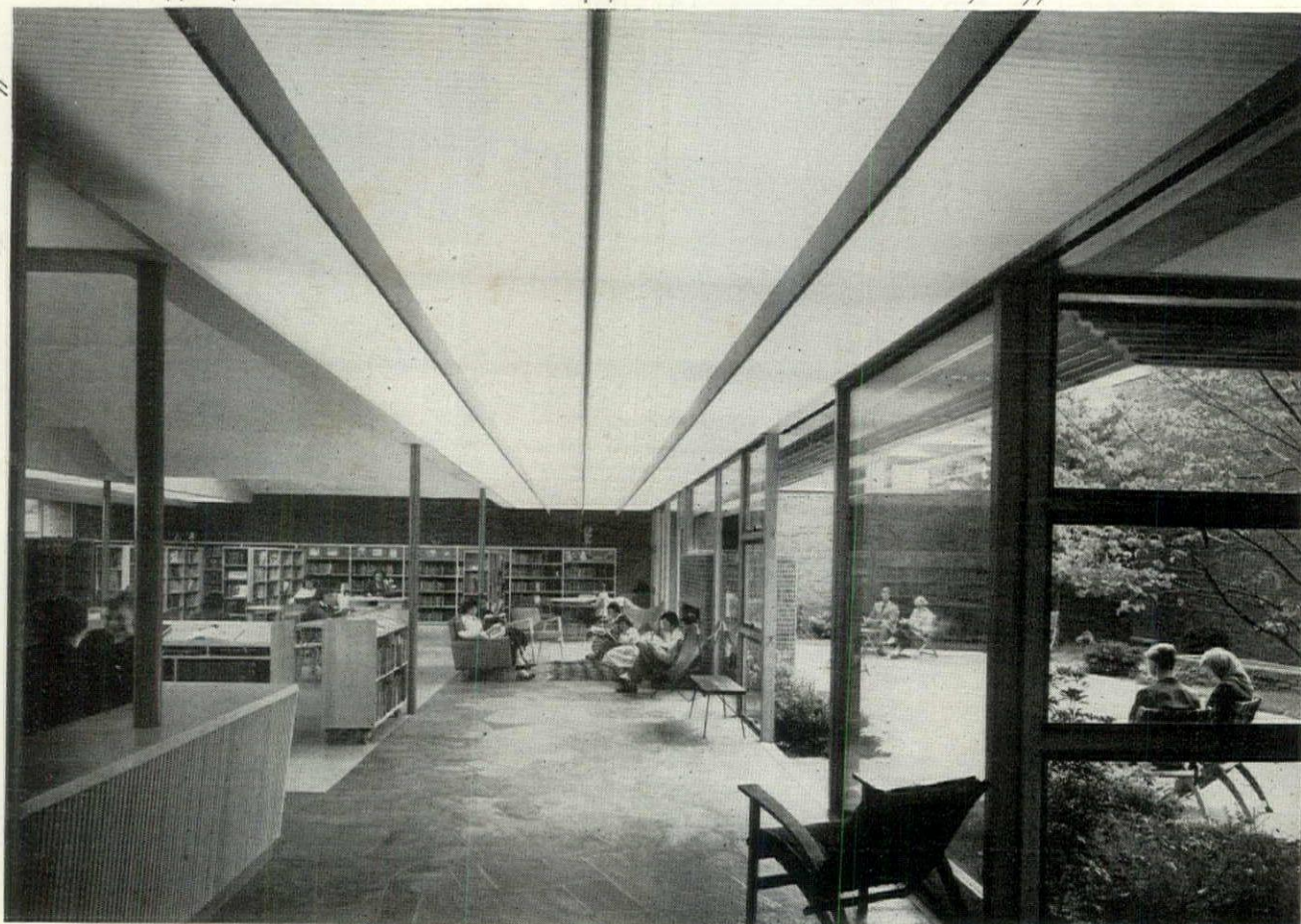
View of reading room showing construction of luminous ceiling
