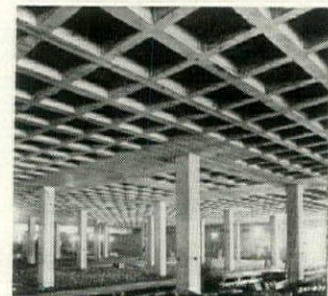
Meyer Steelform Construction uses little steel, provides long spans, maximum manufacturing area free of columns.
