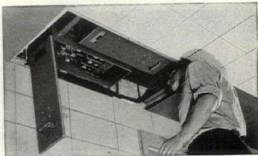
Dark runs on either side of the ceiling mark paths of bus duct in Electrical Engineering Building.
