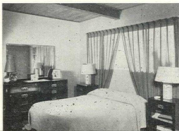
Interior photos show attractive stained ceiling made of kiln-dried, tongue and groove 2" x 6" planks and 6" by 8" beams.
