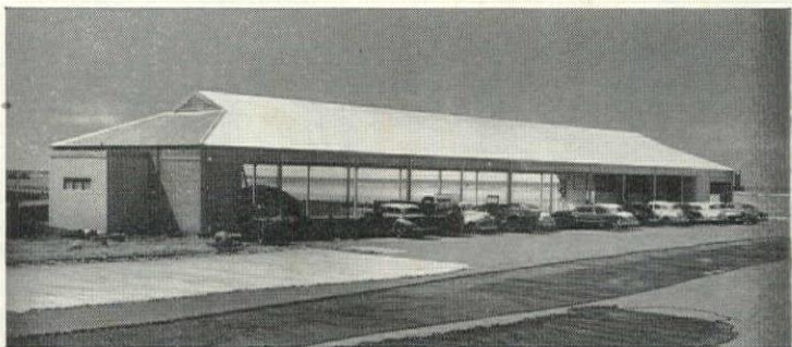
THIS FISH NET SHED, covered with Kaiser Aluminum Roofing, is designed for a seaside location in a hot climate. The roof is highly resistant to the corrosive action of salt spray from the nearby ocean because Kaiser Aluminum Roofing is solid aluminum—not clad or veneered. And Kaiser Aluminum Roofing reflects up to 60 per cent of the sun's rays, which means a reasonably uniform, cool temperature under the shed.
