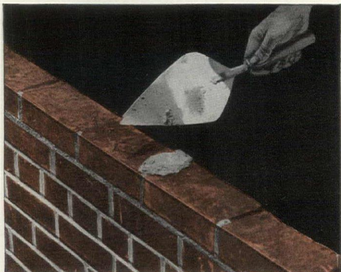
Slushing does not properly fill the voids in the head joints.
