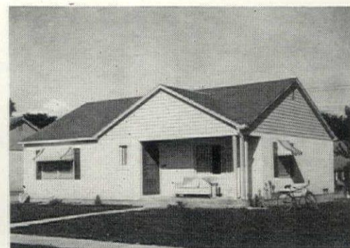
Bonforte Construction Co., biggest defense builder at Colorado Springs, erects stucco homes.
