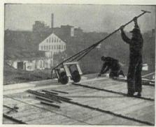
Quickly Positioned . . . unskilled labor casily handles FLEXICORE with simple two-wheeled tool . . .
