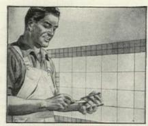
Waterproof adhesive applied to back of the tile insures life-time bond with foundation.
