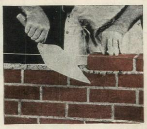
two photographs above show a good comparative test for plasticity—hence for bond. Try this with Brixment mortar!
