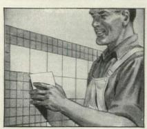
Formed edges of tile fit foundation sheet grooves which are designed to take all tile
