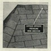
Plan courses so nails at ridge are covered by at least 1" of overlying ridge shingle. Last course of roof shingles may be turned over or trimmed even with ridge. Shingles at hips should be trimmed even with hip line. For cover shingles on ridges and hips, use Master-Bilts cut in thirds and trimmed to edges of "cutouts". Laywith butts exposed 5" to weather. Place nails 1½" from each side, not over 6" from butts. On ridges always expose opposite prevailing wind direction.
