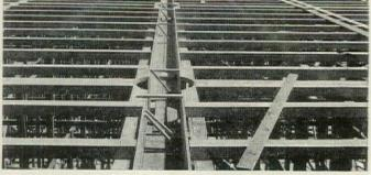
Simple open wood centering is all that is required in Meyer Steelform construction. The centering may be re-used from one floor to another, as can Meyer Steelforms. This eliminates extra lumber costs, saves time.
