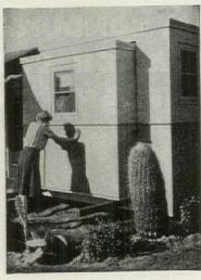
COMPLETE HOUSE (left) may be placed on eleven standard building blocks or a continuous foundation wall. Bedroom wings (right) telescope easily for transportation to a new location. Extended, the wings create two enclosed bedrooms capable of sleeping a family of four, plus storage space.
