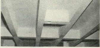
Fire-resistive construction shown in a close-up view. Notice the finished character of ceiling joists built with Meyer Steelforms. Concrete joists can be left exposed or a flat ceiling can be attached.
