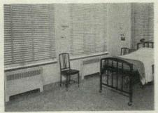
Simple to Keep Clean... Easily removable enclosure front makes heating unit conveniently accessible. Smooth non-porous copper surface is not a catch-all for germ-laden lint and dust.
