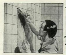
Squeegee removes excess grout; joints are pointed; tiles cleaned with sponge and fine
