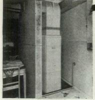
Compact Janitrol Forced Warm Air Furnace fits in "closet-size" space. Unit only occupies 18" by 27" floor area.
