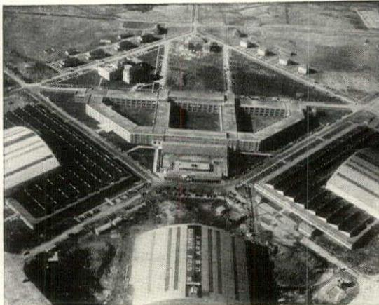
★★★ CHANUTE FIELD, the nation's foremost air training center. ZONOLITE CONCRETE used for insulating roof fill over almost four acres of concrete roof deck—and for all saddles and cant strips. Photo courtesy of U. S. Army Air Corps. ★★★
