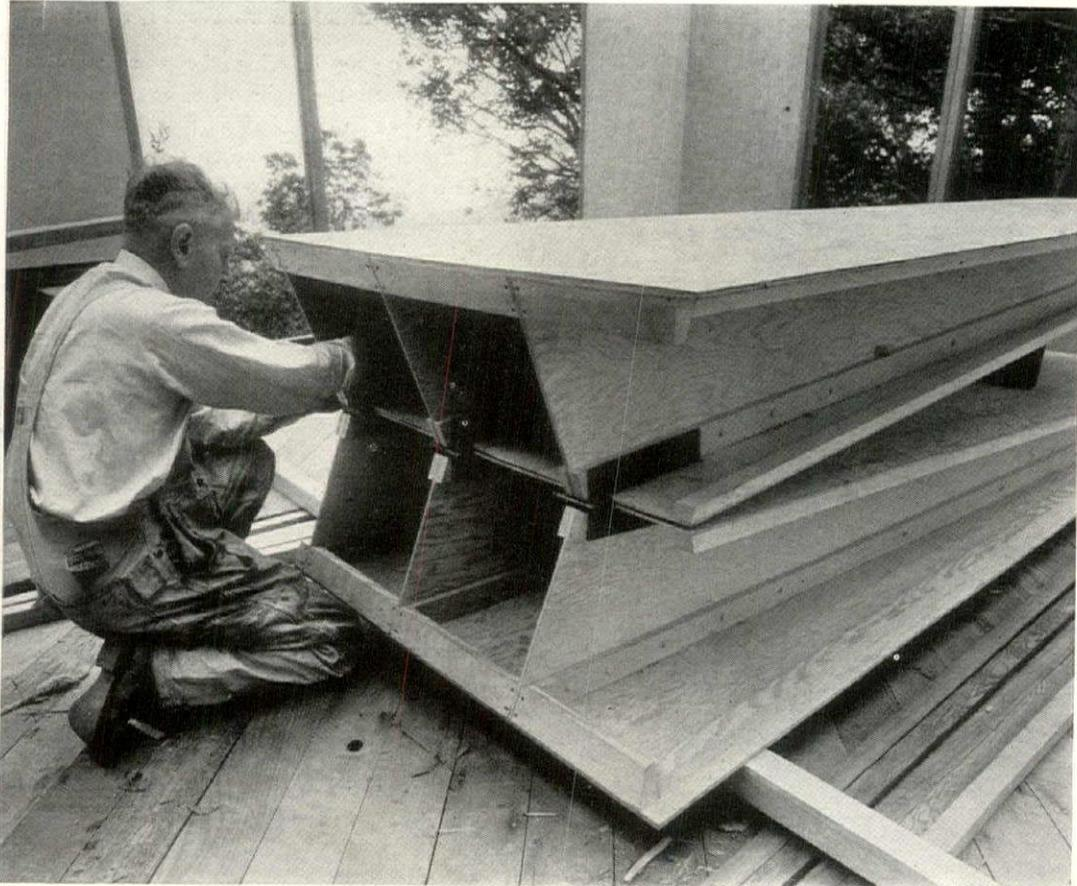
In the photograph above the simple and ingenious design of the folding roof can be studied. The entire tensile stress developed when the roof is loaded is taken by the hinges, which are simple loose pin butts with four steel straps welded on.
