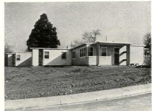
**Pease Woodwork Co., Inc., Turrill St., Cincinnati, Ohio,** prefabricated its first Peaseway House in April 1940 based upon previous experience in selling building materials by mail. Construction system uses wall-length exterior panels, room-length floor panels. Factory in Hamilton, Ohio, equipped with moving assembly lines, has produced 500 houses to date. Capacity of 1200 within 90 days.
