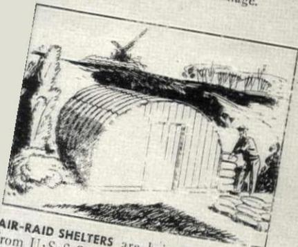
**AIR-RAID SHELTERS** are being made from U·S·S Sectional Plate Arches. These are strong and can be quickly erected with ordinary labor.
