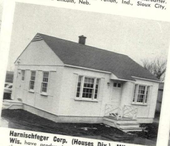
**Harnischfeger Corp. (Houses Div.), Milwaukee, Wis.** have produced more than 1,000 steel prefabs since 1936, recently switched to plywood to meet defense requirements (see above). Capacity, 1,200 in 90 days, 750 a month thereafter. Harnischfeger has supplied 530 units for 3 defense projects.
