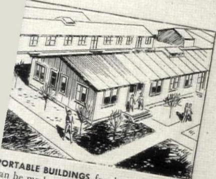
**PORTABLE BUILDINGS** for the fighting forces can be made of U·S·S Steel Sheets and insulated to keep out heat and cold.
