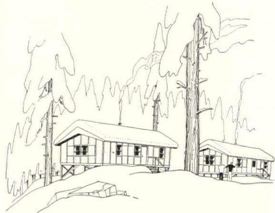
The system may be applied to houses as well as larger structures. At the left is a two-bedroom scheme, well planned for privacy and convenience. The sketch of the snow-covered buildings was included to suggest the strength of the roof, which, by increasing the thickness of the plywood sections, will carry loads in excess of 100 pounds per square foot. Also to be noted is the manner in which the buildings may be adapted to irregular sites.
