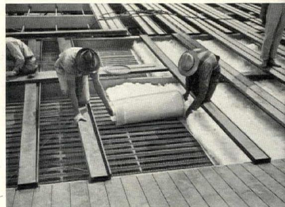
**ROOF CONSTRUCTION.** Above you see roof nearing completion. Workmen are unrolling Fiberglas blankets. These in turn are covered by Truscon Ferrobord Steeldeck, Fiberglas roof-deck insulation, and finally by waterproof roof material.
