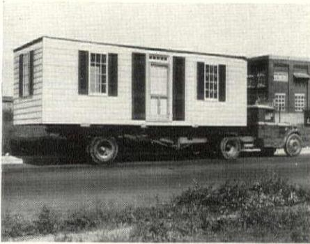
1937. Architect John Whelan, in Washington, D. C., developed an experimental mobile, 2-part house, sheathed in copper-crippled to resemble siding. (AF July 1937, p. 53-5).
