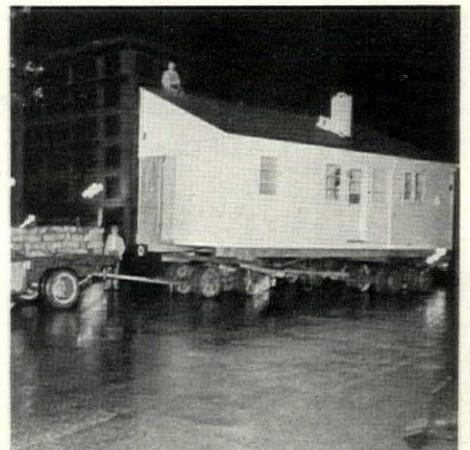
1939. Seattle Architect George W. Stoddard built a number of wood frame and plywood houses indoors in 2 to 3 parts, moved them to the site on trailers. (AF Apr. 1939, p. 286).
