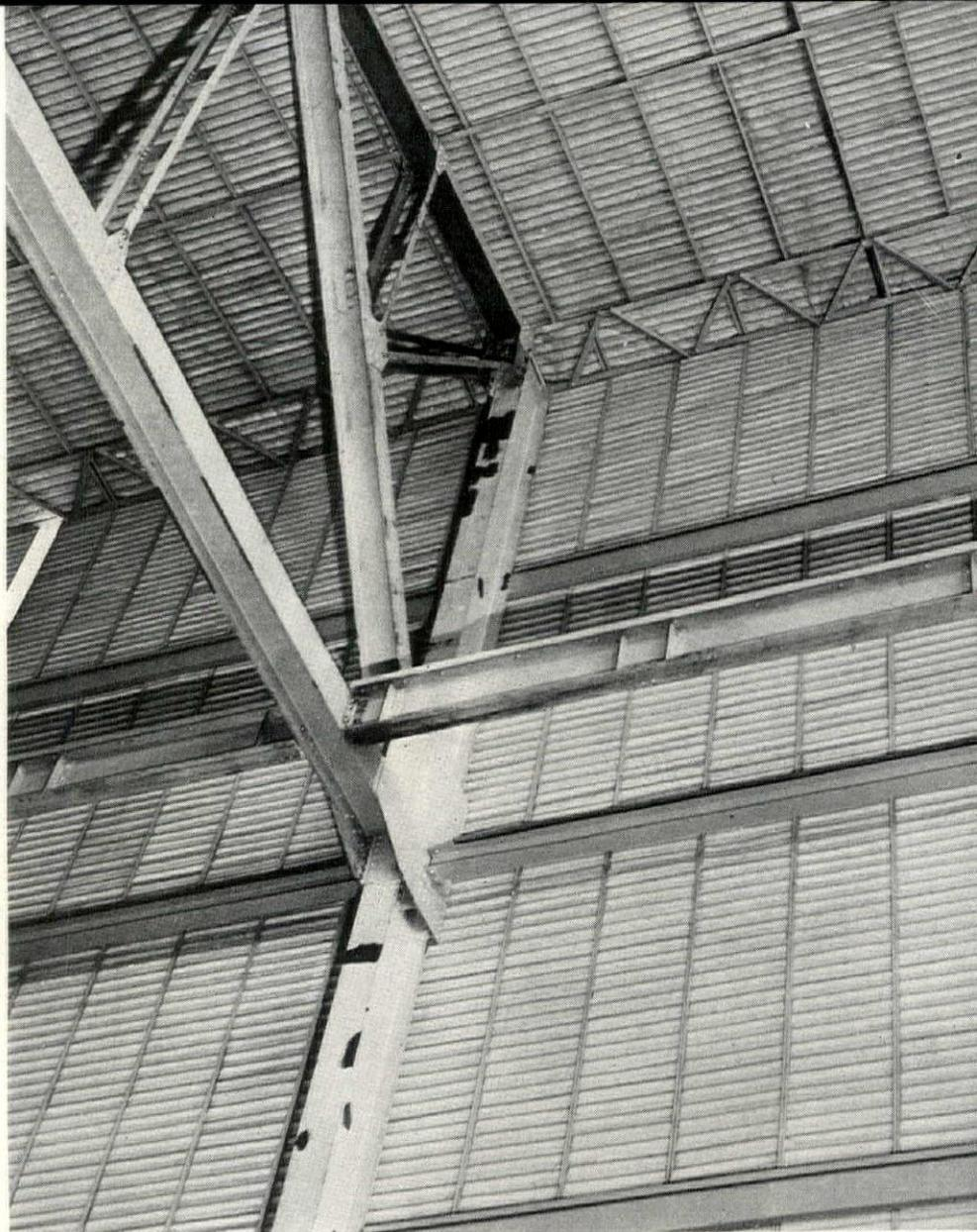
The illustration above shows the interior finish which is standard throughout the plant: a layer of expanded metal lath, through which is seen the core of highly
