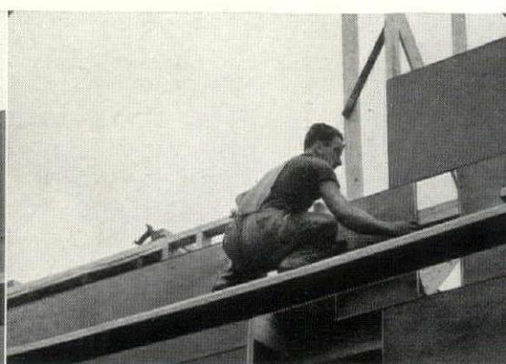
3 Eliminates mis-nailing—studs are in plain view always—don't have to be exactly centered.
