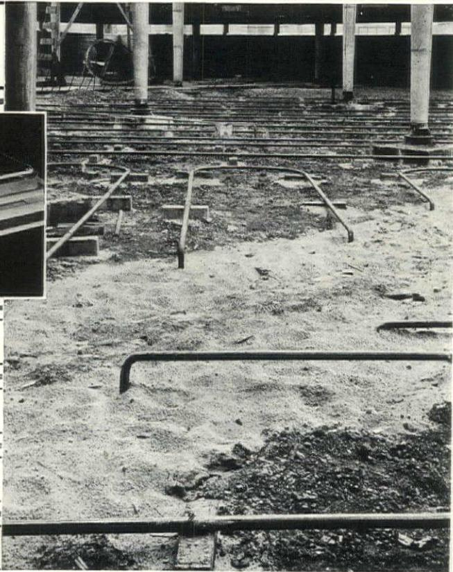
In heating, also, the modern office building of S. C. Johnson & Son, Inc., strikes a unique note. Steam pipes of Byers Wrought Iron imbedded in the floor combine with tempered ventilating air to warm the structure.
