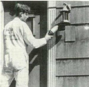
**FOR SIDE WALLS** in present homes, Gimco insulation experts make small, easily refinished openings in outside and blow Gimco between walls.
