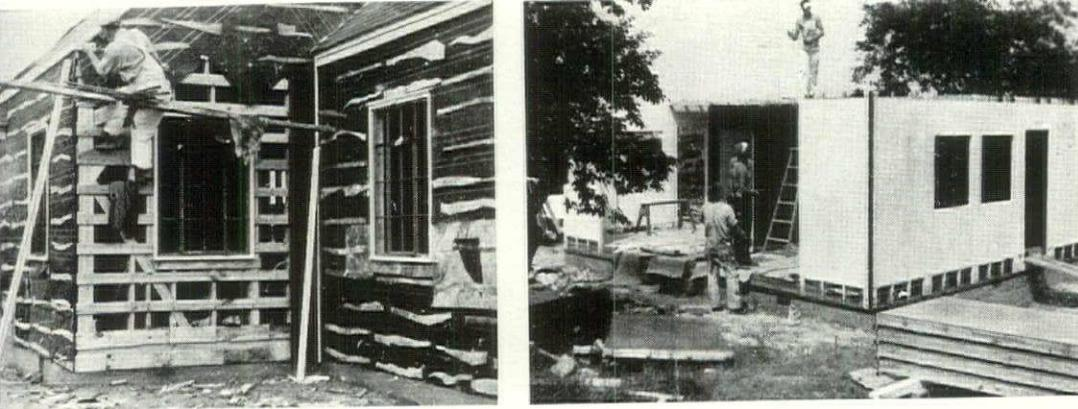
Ex-ray of the conventional houses' frame construction is presented above, left. Asphalt shingles were applied to shingle battens, separated only by a layer of tar paper. More substantial are the cross-braced and insulated plywood panels, right. Taken at 1:30 p. m., the picture indicates the speed with which the prefabricated houses were erected—seven hours earlier only the poured concrete foundations were in place.
