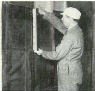
**IN SIDE WALLS** of unfinished homes, Gimco Bats fit standard spaced studding. Easily cut to fit any irregular-shaped spaces.
