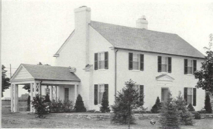
ABOVE—Air conditioned Manor House designed by M. R. Evans of Lancaster, Pa., for the Lancaster Real Estate Board as a model home. All exterior walls are insulated with full inch Armstrong's Temlok.
