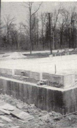
ft. foundation walls waterproofed with emulsified asphalt. ght, The I-beams in place for floor construction.
