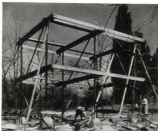
LALLY COLUMNS AND BUILT-UP AND NOTCHED BEAMS
