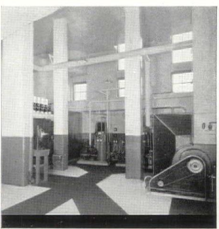
● A view of the fan room in the Sheboygan County Court House, showing parts of the court room and jail systems, with their automatic controls.
