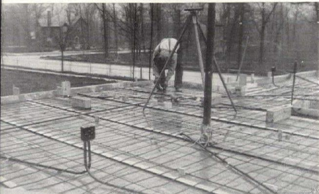
reinforcing floor with 1/4 steel rods, at intervals of 6 in. on center.
