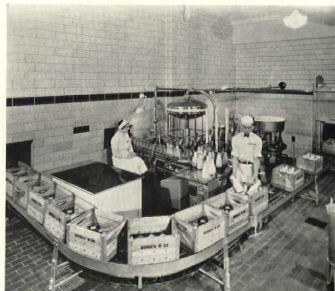
Vacuum bottle filler which caps 60 quarts of milk per minute. Conveyor leads to milk chill room
