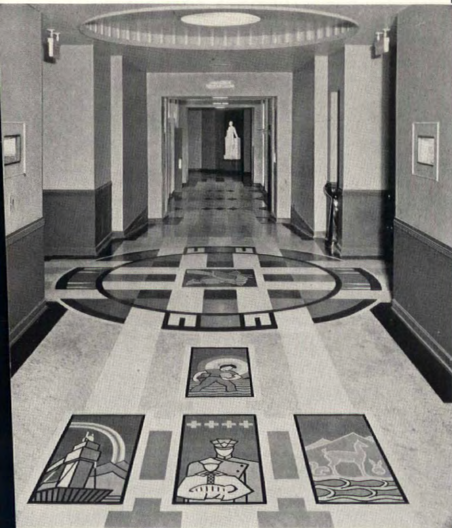
In the Illinois Host Building at the "Century of Progress" this fine mosaic floor of Armstrong's Linoleum showed hardly any wear after months of heavy traffic. C. Herrick Hammond, F.A.I.A., Supervising Architect
