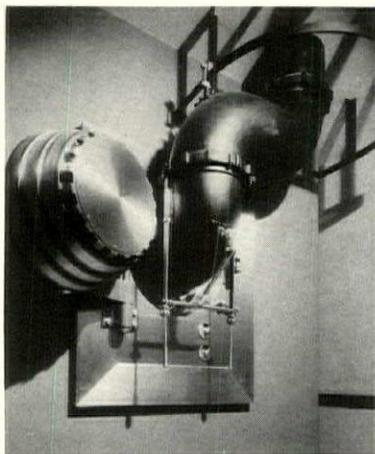
Above is the conditioned air supply to the vault. It may be removed at will. Below is a typical fan supplying one of the main ducts
