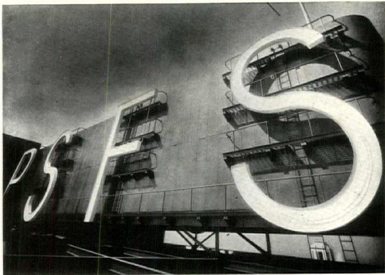
The steel background for the huge electric sign on the roof of the office portion of the building conceals part of the air conditioning equipment shown at the left. The letters of the sign are 27 ft. high and 15 ft. wide. They are formed with a white porcelain enamel face and are lighted by red neon tubes. The background of the sign is painted a cobalt blue
