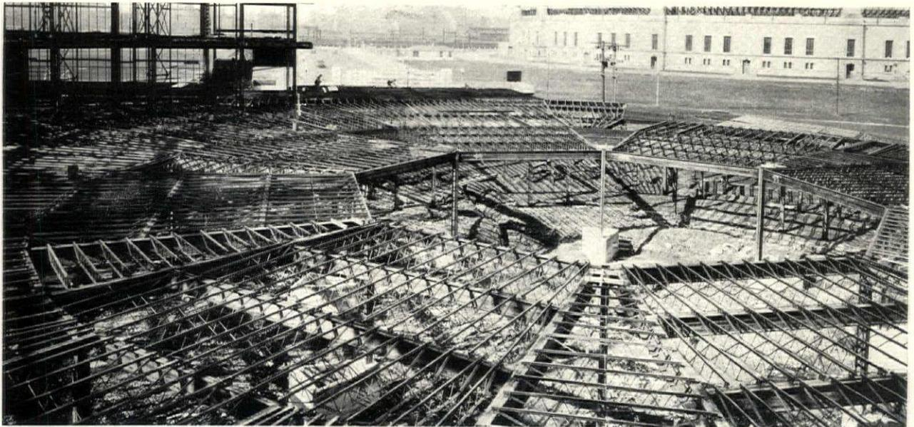
A view of the north terrace and central court during the process of construction. It shows the method of steel framing employed throughout the building, as well as the concrete footings which serve as pile caps
