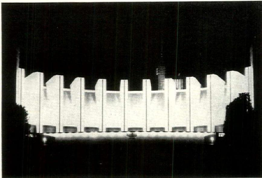
Two methods employed in lighting the Hall of Science. At the left is a night view of the north facade. The twelve pylons are illuminated. The twelve pylons are illuminated by means of neon tubes complemented by floodlights at the base. Below is a view of the interior lighting in the Great Hall where the neon tubes are concealed by a system of suspended covers
