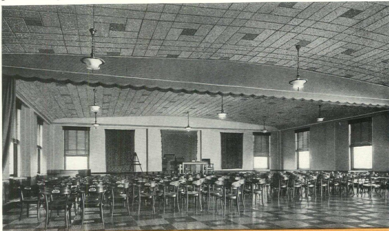
THIS AUDITORIUM CEILING has been treated with Armstrong's Corkoustic Type C for acoustical correction. Note the pleasing decorative effect secured by combining unpainted and painted panels. Ease of cleaning assures low maintenance costs.
