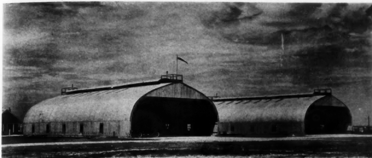
Houston Airport Hangars. Welded Steel Frame, Corrugated Iron Covered, Rigid, Strong, Fireproof and of Moderate Cost
