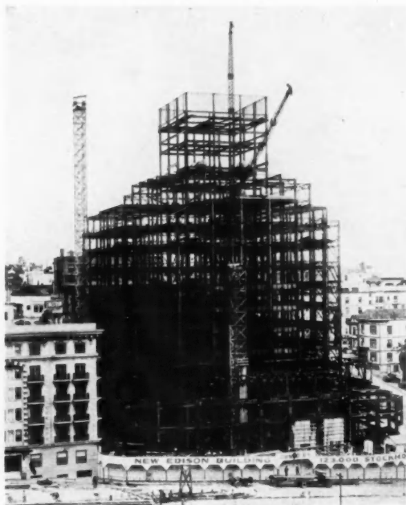
The 3,000-Ton, Shop-Riveted, Field-Welded, Steel Frame of the New Southern California Edison Building, Los Angeles, California
