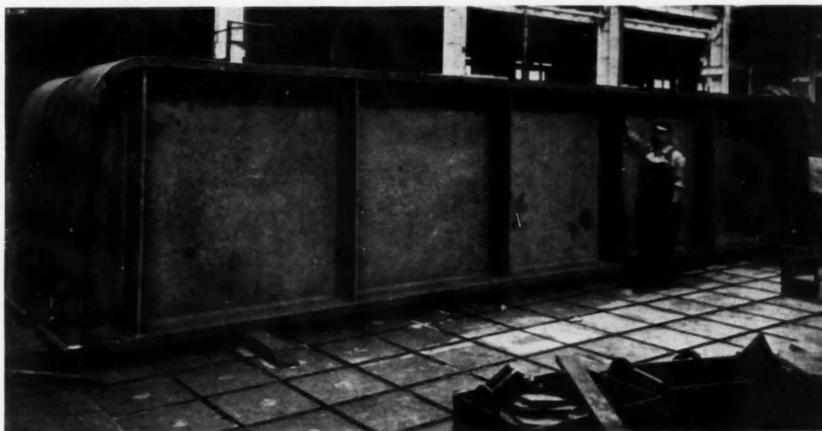
All-Welded Plate Girders to Support the Upper Bearing Bracket Form 19,000 KVA Waterwheel Generator. Note Absence of Connection Angles
