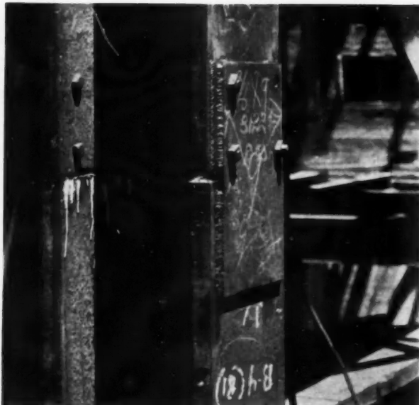
Welded Column Splice, Field Erection Bolts
