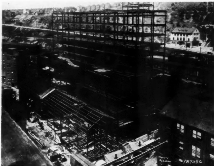
Central Engineering Laboratory of the Westinghouse Electric & Manufacturing Company, East Pittsburgh. 2,000 Tons of All-Welded Steel, 11 Stories High, 222 Feet Long by 120 Feet Wide
