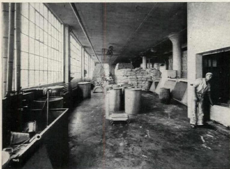
*The floors in many plants and warehouses are continually covered with substances that cause and accelerate disintegration of the concrete. The condition pictured here is commonly observed.*
