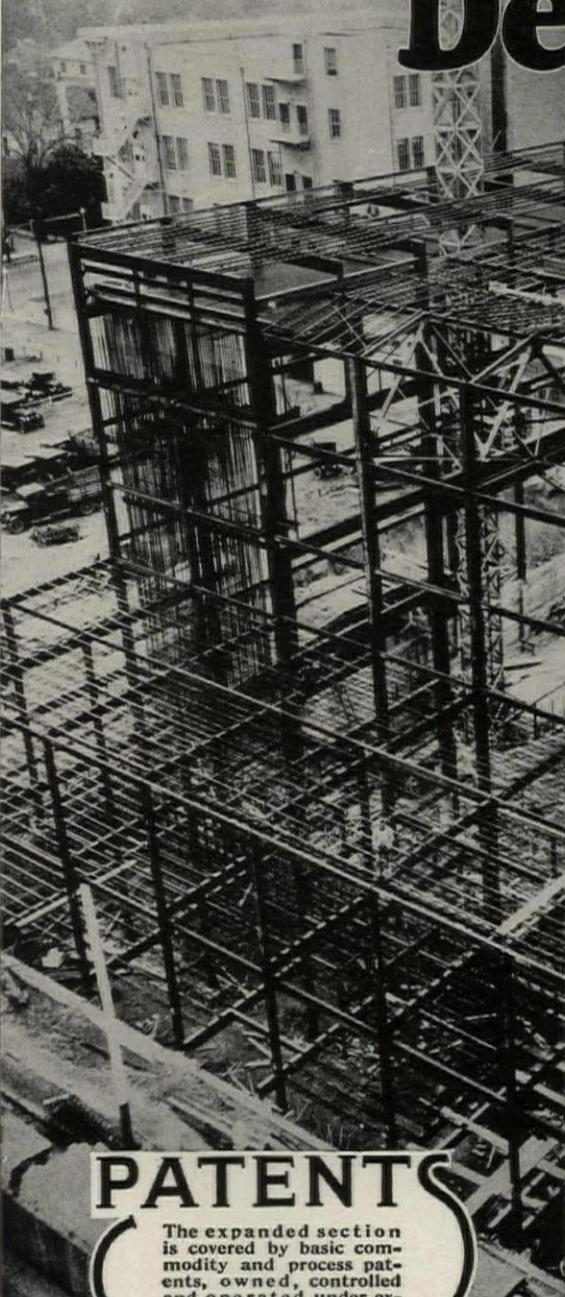
**NO WELDS IN STRESS**—one piece of steel—expanded—without rivets, bolts or welds in shear or tension—these are the features responsible for the rapid gain in Bates-Truss Joist popularity.
