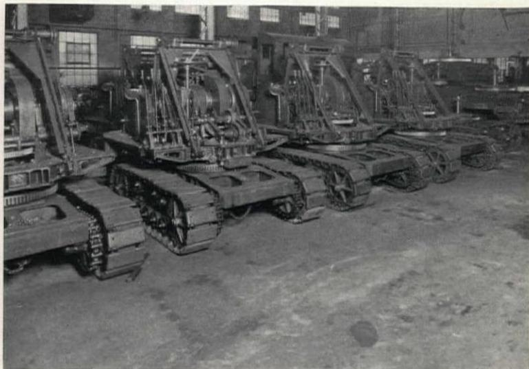
*Abrasive wear from heavy equipment or loaded trucks is at best a severe test. Failure starts at spots where oil drippings have been absorbed and the concrete weakened by the consequent disintegration.*
