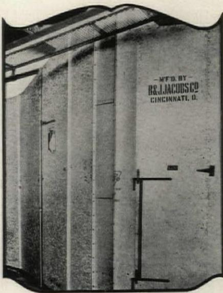
Part of a vast system of ARMCO Ingot Iron ventilating ducts, installed at the Muth Division of the National Biscuit Co., Cincinnati, Ohio. The conditions are abnormal here: steam, heat, and moisture combining to attack the metal.
