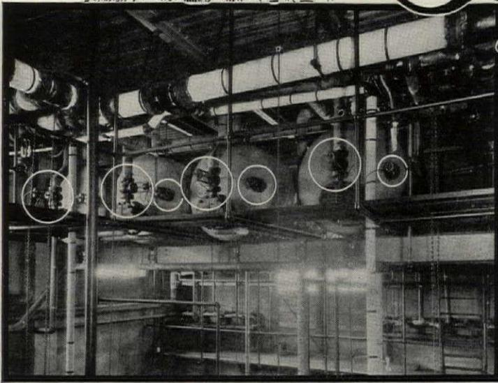
Shown above are four Sylphon Regulators installed on storage tanks in the new Roosevelt School at Des Moines, Iowa. Sylphon Temperature Regulation is an important factor in maintaining an even school-room temperature, and in regulating the brine cooled drinking water system.
