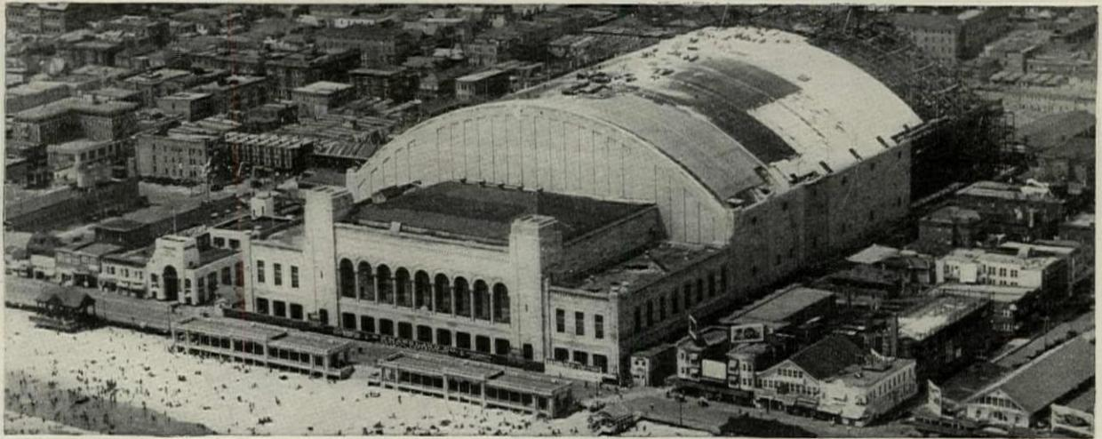
The Convention Hall at Atlantic City has a roof area of 220,000 square feet. The roof deck is of Gypsteel Pre-Cast Gypsum Slabs. Lockwood, Green & Co., Engineers
