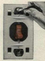
2 Fasten switch to outlet box—no "building-up" necessary.
