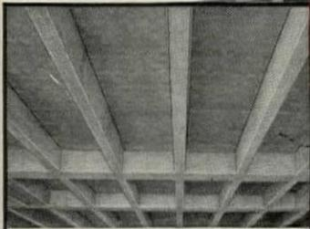
*Note the clean-cut, good-looking joists when Meyer Steelforms are used. Meyer Steelforms are installed and removed by a trained organization. A nominal rental charge based on continued re-use of the sturdy steel forms covers installation and removal.*
