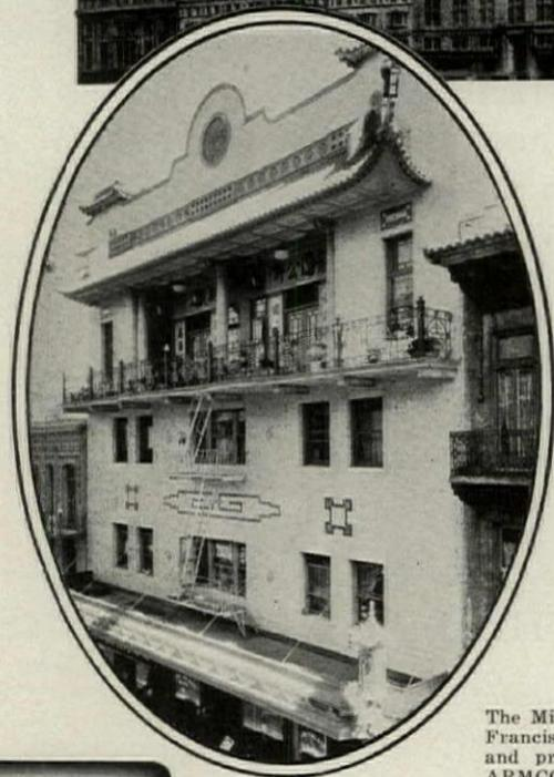
The Ming Yee Building, San Francisco, is well equipped and protected with durable ARMCO Ingot Iron. The architect, Charles E. Rogers, specified pure iron for marquises, ventilators, ornaments and metal tile because of its pronounced workability and longevity.
