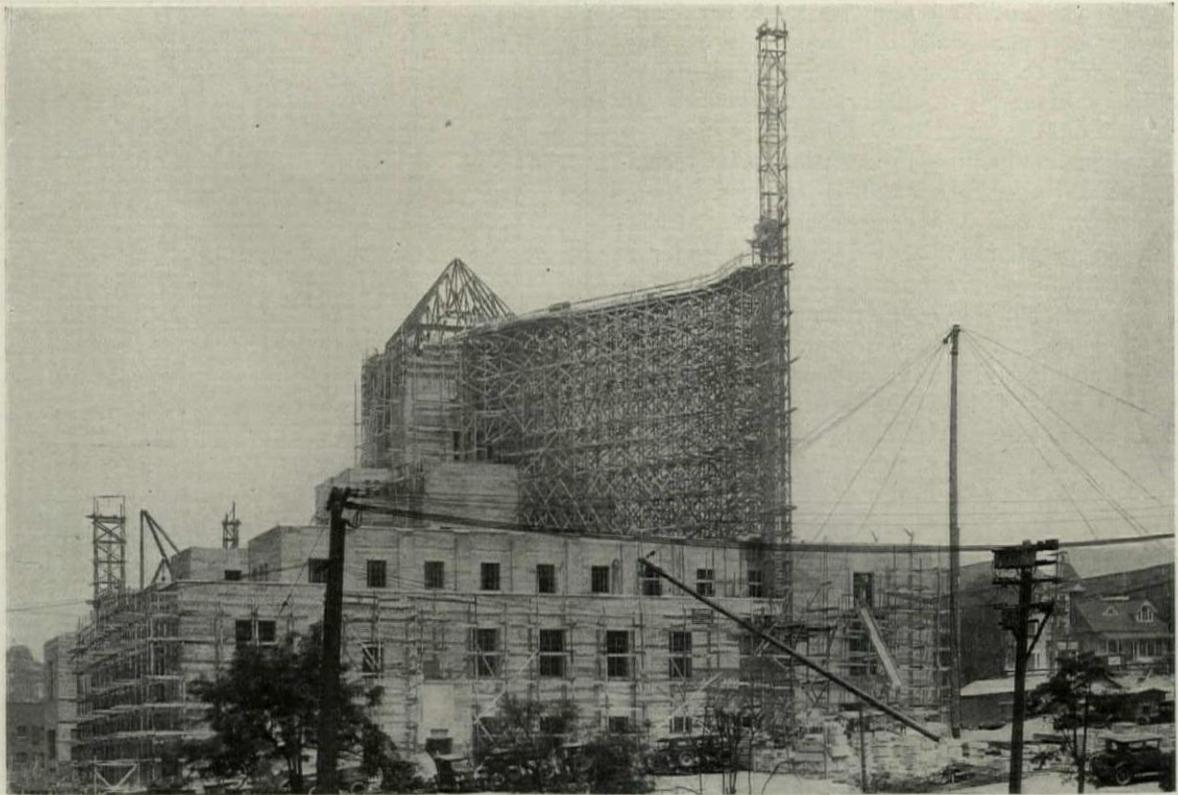
Los Angeles Public Library, Under Construction, Showing the Use of Poured Concrete for Exterior Walls
