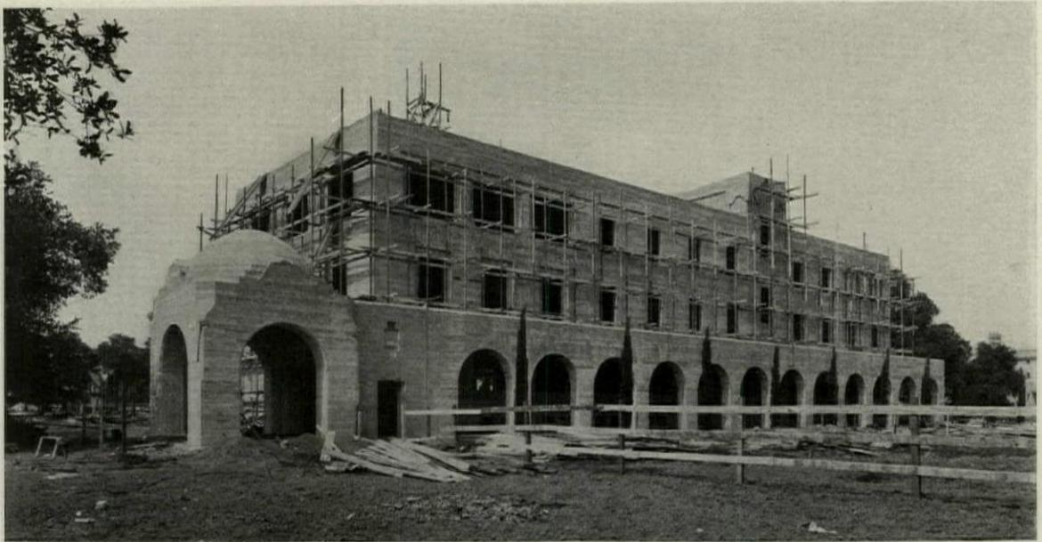
The Biology Building, California Institute of Technology, Illustrates a Design Particularly Suited to Reinforced Concrete. The Wall Surfaces Were Later Stuccoed
