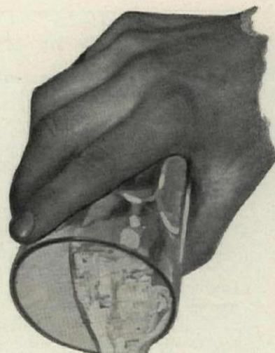
*Being cellular in structure, not fibrous, Armstrong's Corkboard will not absorb or hold water. It can be drenched with water, or completely submerged, or even boiled, and its granules will remain perfectly dry inside*
