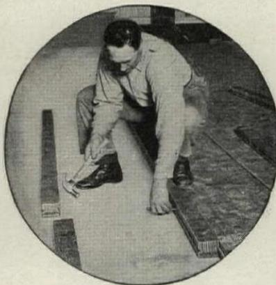
The hazard of splinters—ever present in ordinary wood flooring—is eliminated when Bloxonend is used. The tough end-grain forms the wearing surface. This surface (2½ in. thick) is firm and fast, yet affords cushion-like resiliency. It is handsome, noiseless, lasts a lifetime, stays smooth and provides satisfactory anchorage for apparatus and machines. Write for specifications, descriptive literature and sample.
