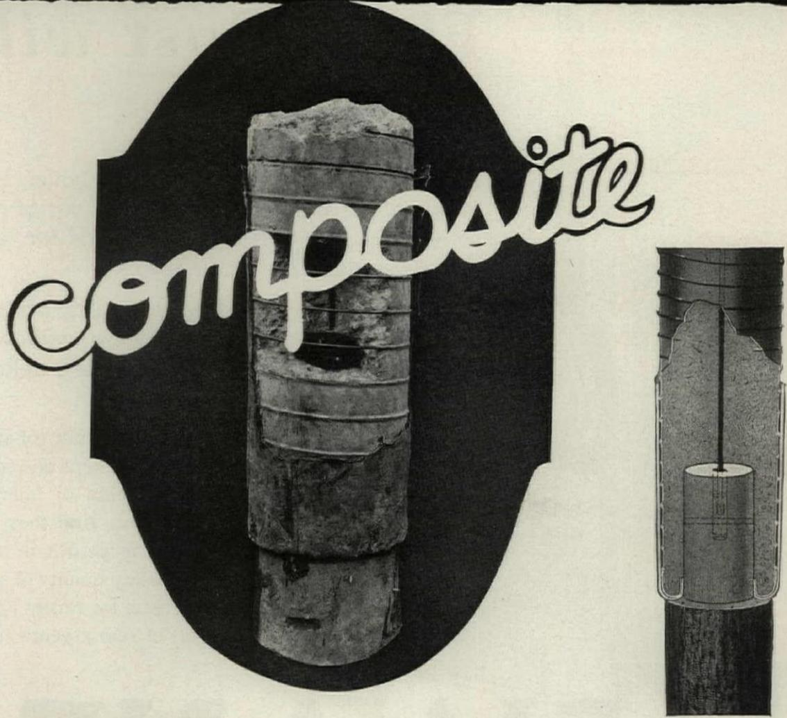
VIRTUALLY a one-piece pile—that is the result obtained by the Raymond Method of joining the timber to the concrete in this type of long pile. It is as perfect in the ground as on paper, as this cut-away section demonstrates.
