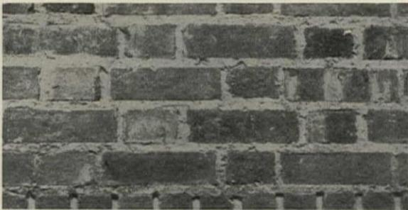
Rough Flush Joints, of Coarse, Dry Mortar Cannot Be Expected to Be Rain-tight in Exposed Locations
