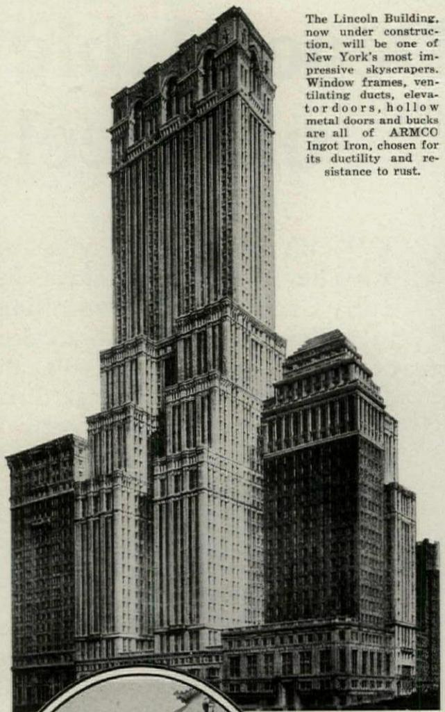
The Lincoln Building, now under construction, will be one of New York's most impressive skyscrapers. Window frames, ventilating ducts, elevator doors, hollow metal doors and bucks are all of ARMCO Ingot Iron, chosen for its ductility and resistance to rust.
