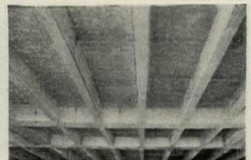
Note the clean-cut, good-looking joists when Meyer Steelforms are used. Meyer Steelforms are installed and removed by a trained organization. A nominal rental charge based on continued re-use of the sturdy steel forms covers installation and removal.
